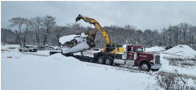
Photo 3- Loading UST-3 for transport.
