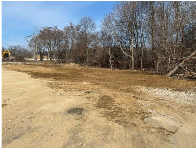
Photo 3 – View of backfilled and graded UST-2/UST-3 area.
