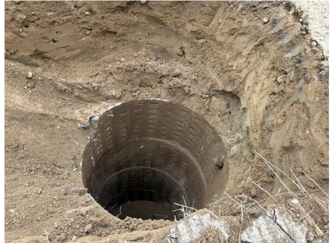
Photo 2 – Cess-6B structure with the concrete dome removed and ready for backfill.
