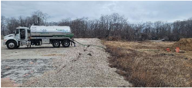
Photo 1 – Clearbrook vacuum truck pumping out liquids from septic tank structures (typical).
