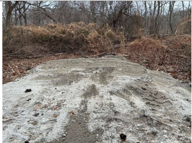
Photo 4 – Backfilled Pit-38 with RCA.
