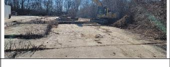
Photo 4 – Removal of concrete slab and concrete cover from septic tank Cess-7A.
