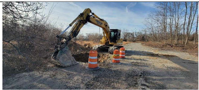
Photo 2- Excavation of formerly backfilled catch basin structure DW-7
