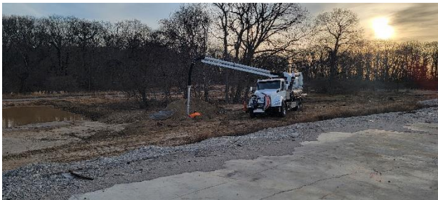
Photo 1 – Cleaning of Cess-12 with guzzler (vactor) truck.
