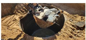
Photo 7 – Central portion of P-7/8 where concrete sump structure was removed. Area was excavated additional 4-5ft (total of 13ft below surface) before collecting endpoint sample.
