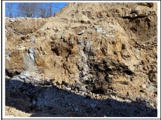
Photo 9 – Pocket of dark soil removed from NW corner of Pit-7/8 excavation.
