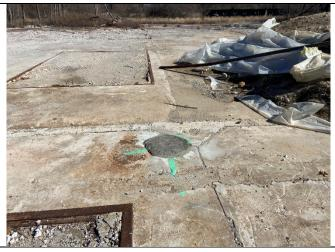
Photo 10 – Example of concreted floor drain (FD-7).
