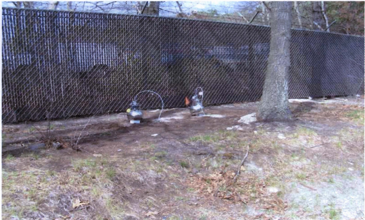
Photograph 1: View of soil vapor points 1S and 1D. Date photo taken: 4/25/2006
