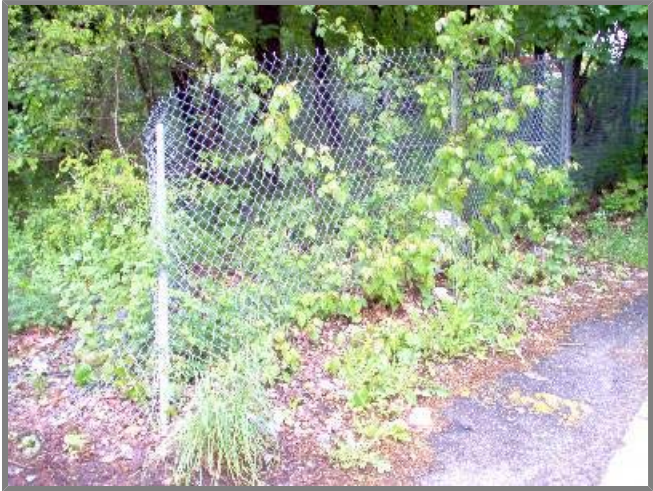
Photo left. Liberty Industrial site, broken gate.
