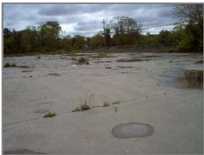
Photo left. Liberty Industrial site.
