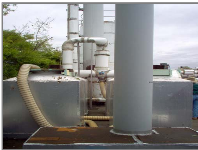
Photo left. Towers and tank. Descriptions from front to back: air discharge tower, air tower from top of air stripper to heater, air stripping tower, and water intake tank.
