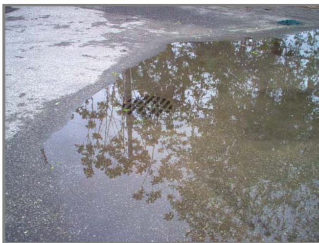
Photo left. Plugged drain in front of the plant.
