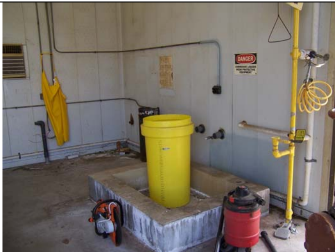
Secondary containment within the GW treatment building
