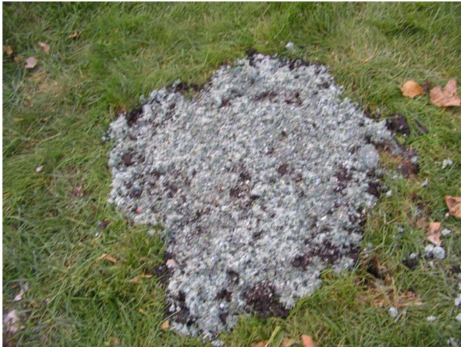
Photograph 10: Grass seeded following well abandonment and manhole removal.
