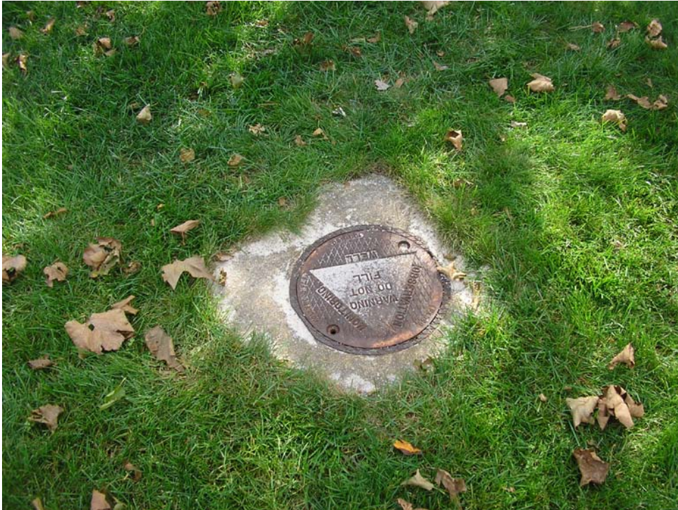
Photograph 9: Well in grass prior to abandonment.
