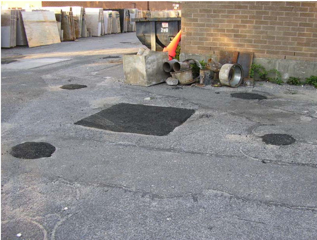
Photograph 6: Asphalt patched.
