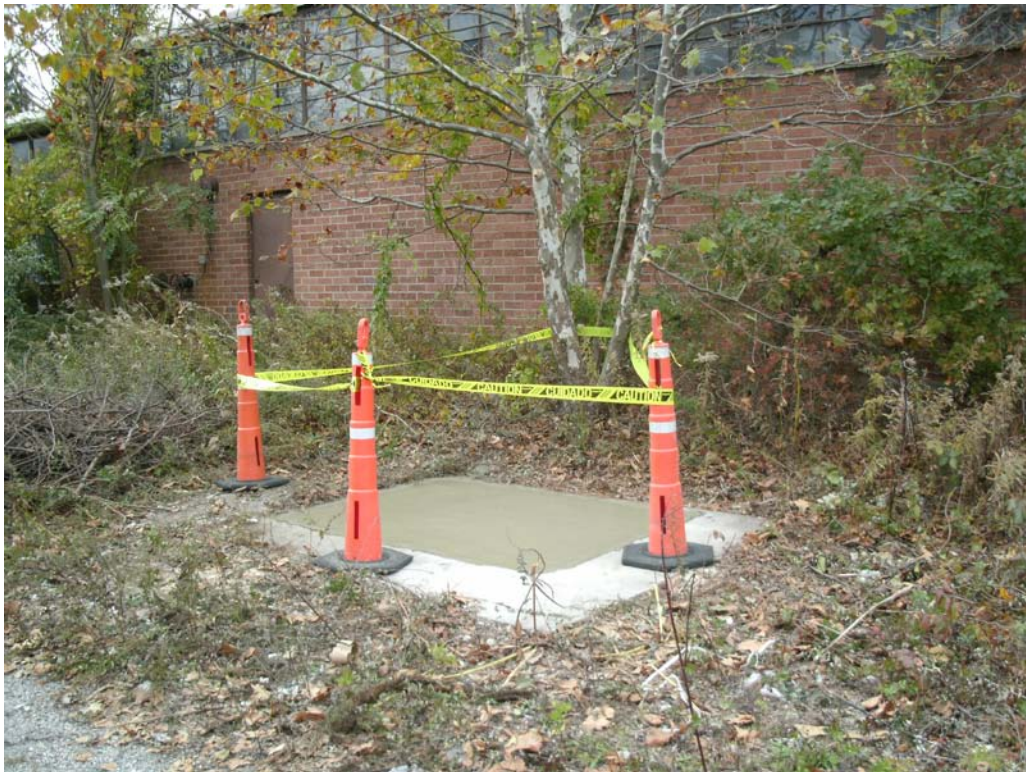
Photograph 8: Off-site pumping well vault following well abandonment.
