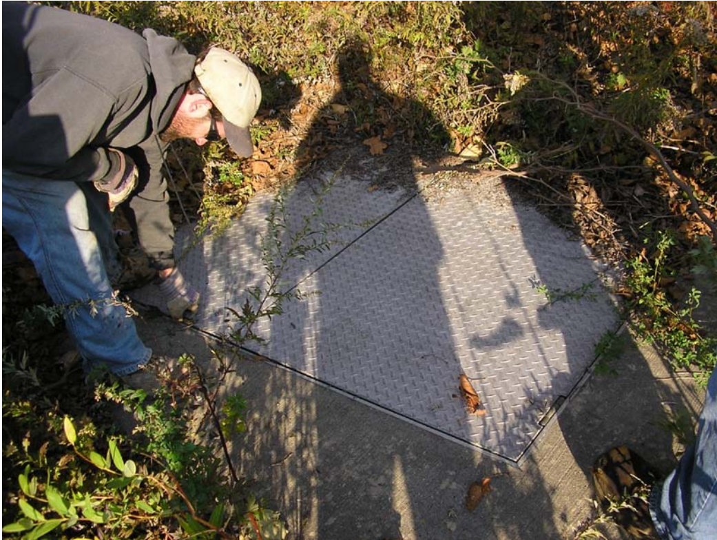
Photograph 7: Off-site pumping well vault.
