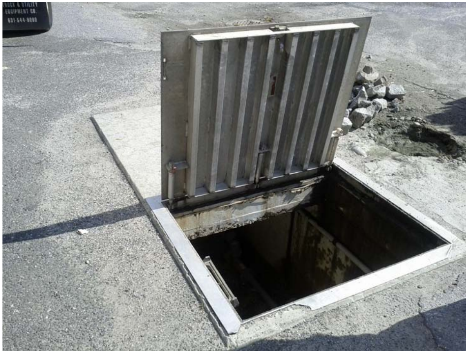
Photograph 2: Well vault for on-site pumping well.
