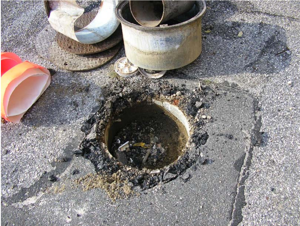
Photograph 5: Removal of manhole covers.
