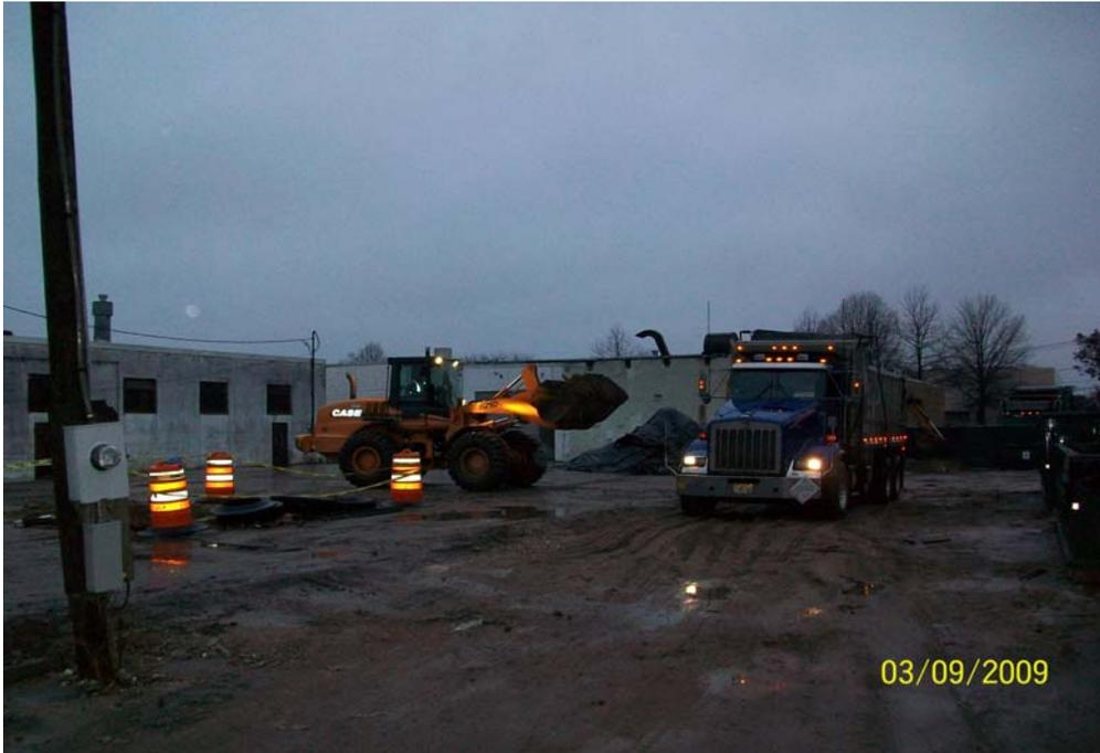
100\_0087.jpg - Front end loader loading hazardous soil into a dump truck.
