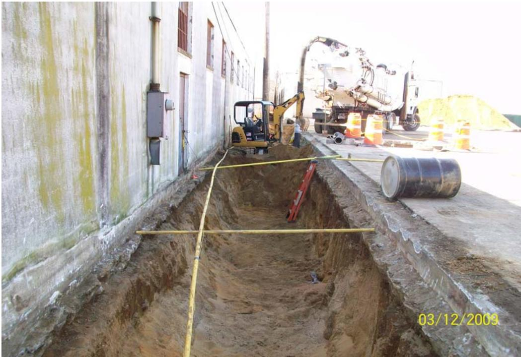
**100\_116.jpg - Excavation of east alleyway, gas line being supported at ~10 intervals.**
