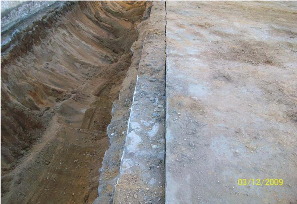
**100\_0111.jpg - Crack separating 50 Dale St. slab from wall.**
