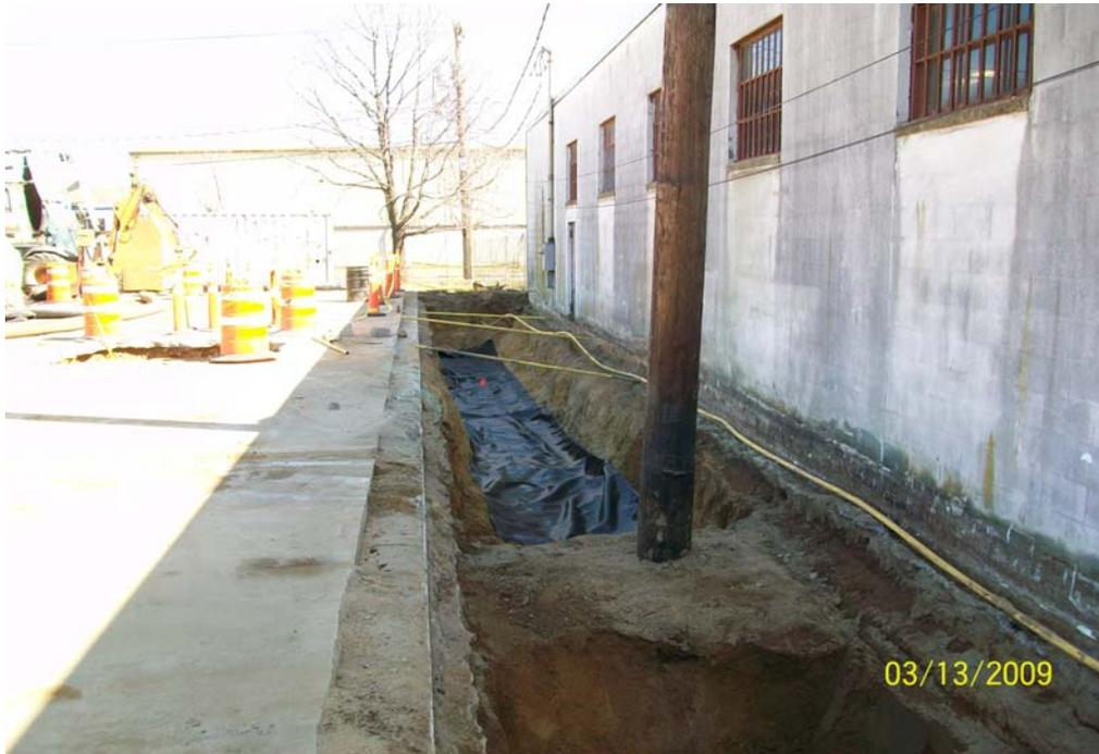
**100\_122.jpg - Filter fabric on east alleyway excavation, looking east.**
