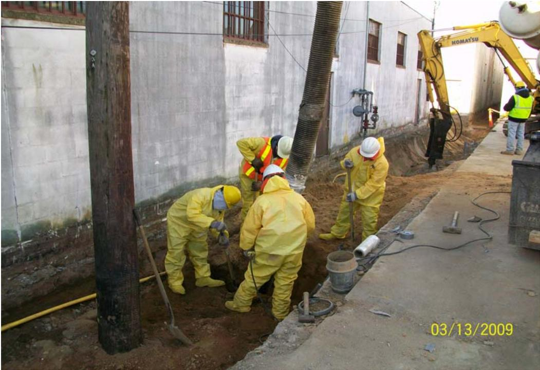
100\_0119.jpg - Excavating east alleyway with vac truck.
