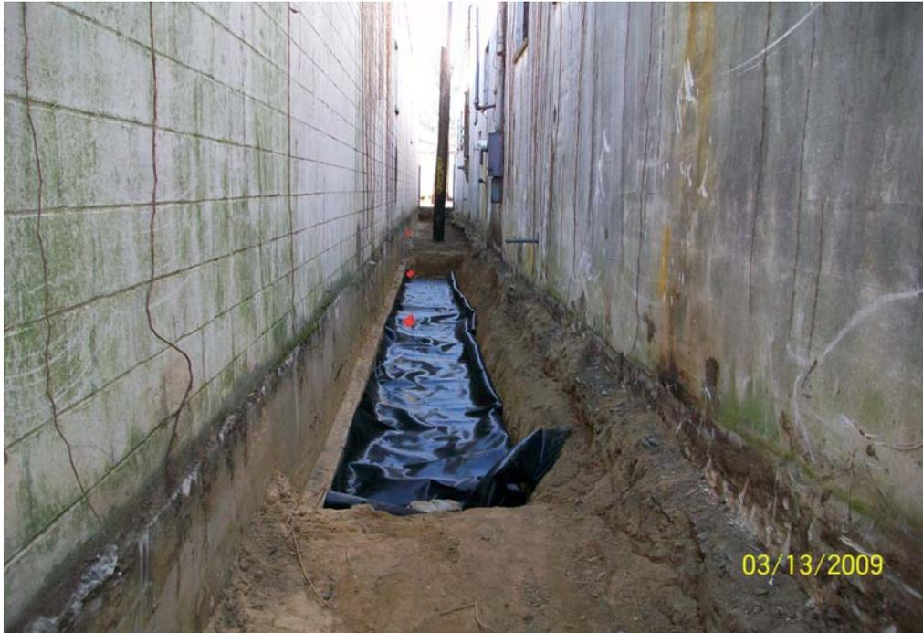
**100\_0120.jpg - Filter fabric on west alleyway excavation. Flags are sample locations, looking west.**
