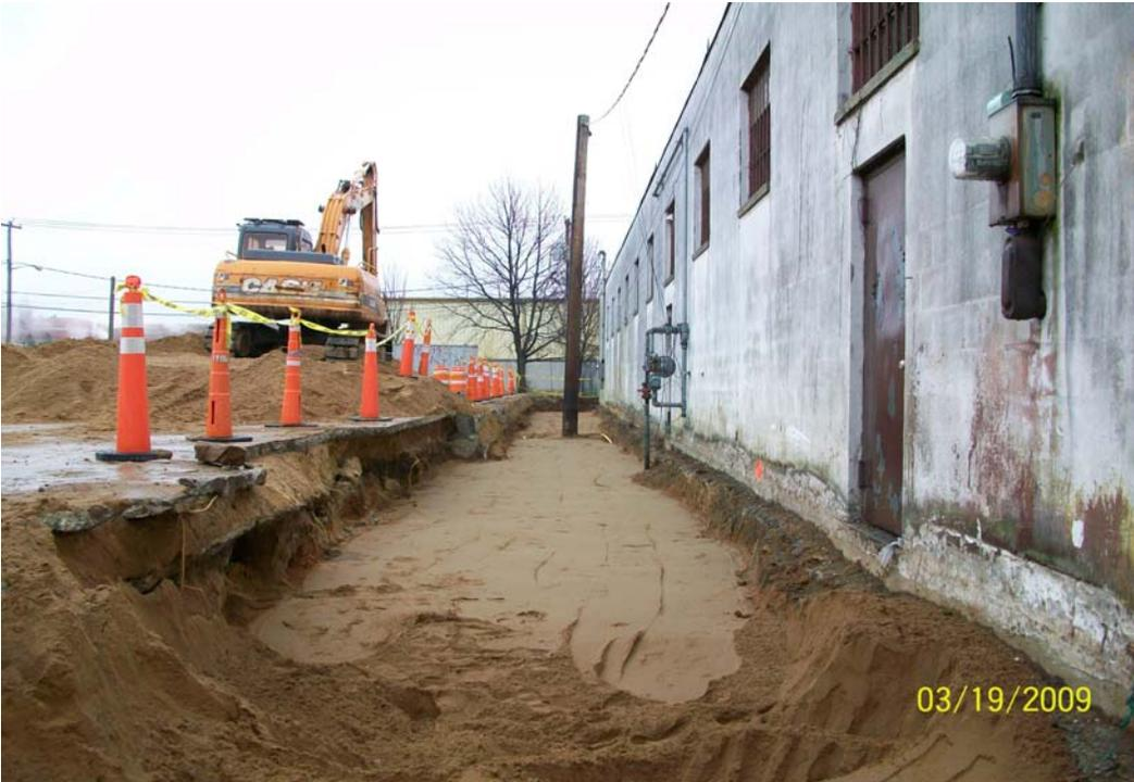
**100\_0036.jpg - Finished backfilling and compacting the east alleyway from the utility pole west.**
