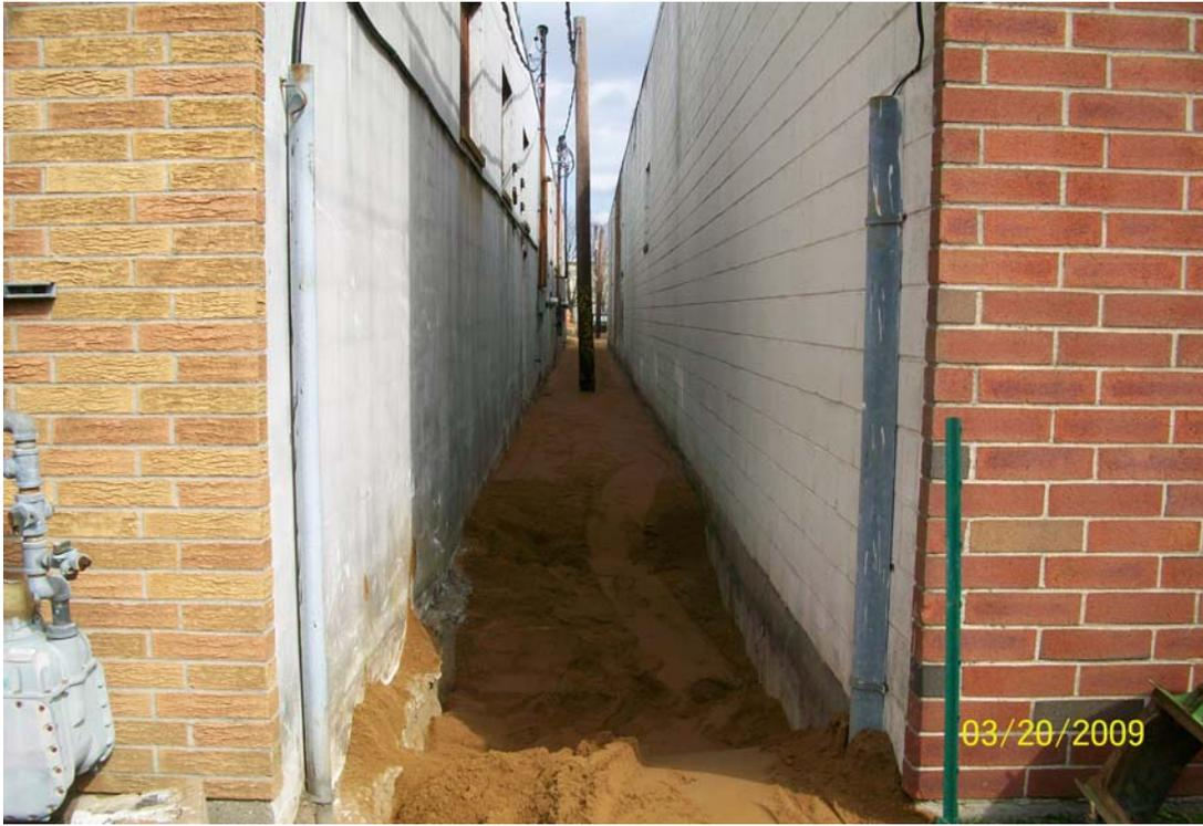
100\_0042.jpg - End of day for backfilling and compacting west alleyway west of utility pole.
