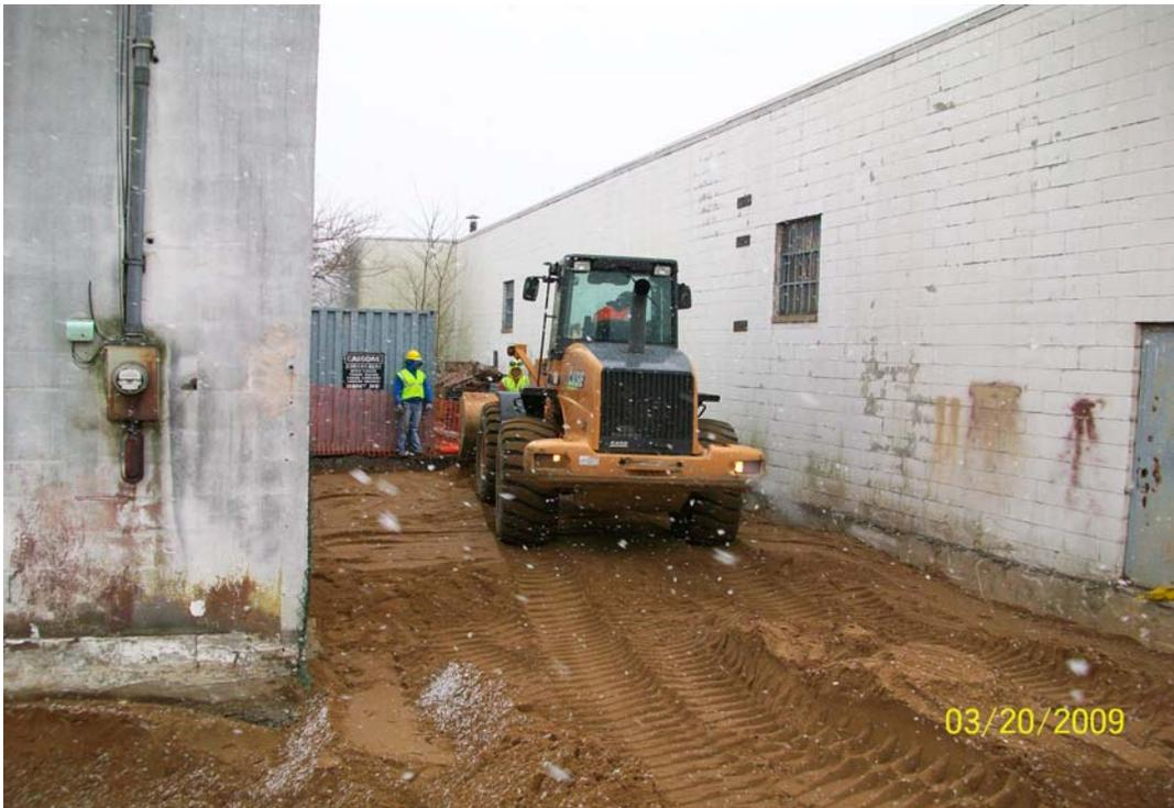
**100\_00139.jpg - Backfilling and compacting south alleyway.**
