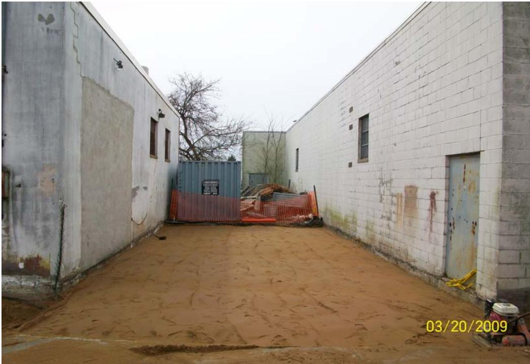
**100\_0041.jpg - Finished backfilling and compacting the south alleyway**
