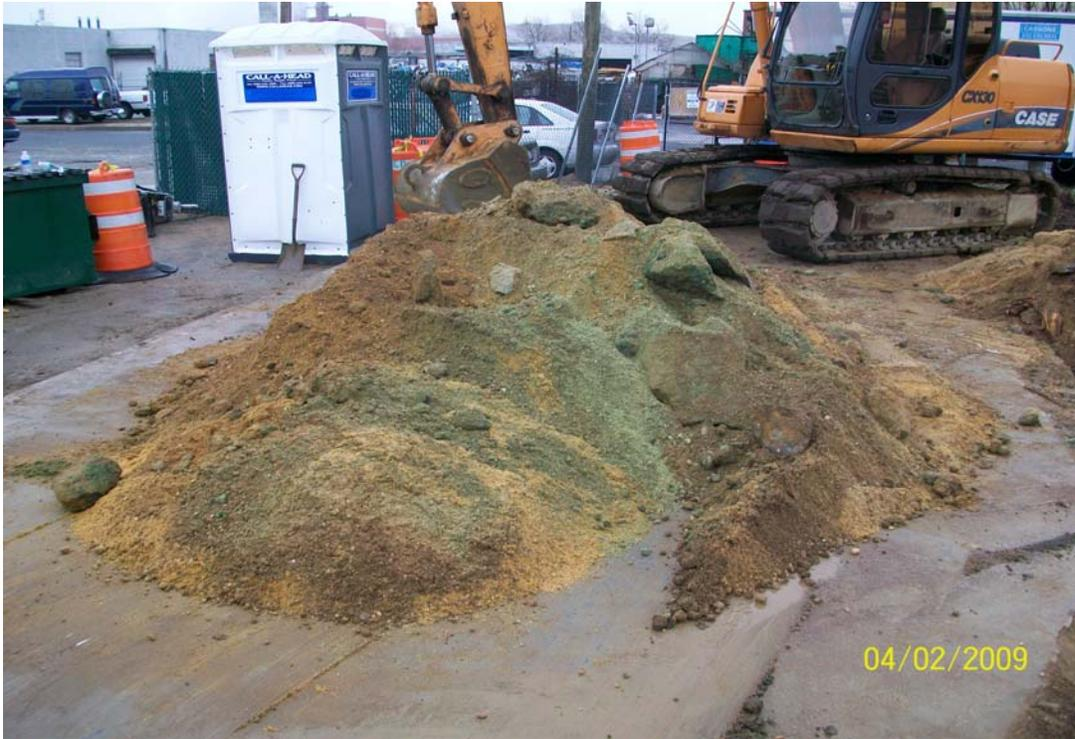
100\_00316.jpg - Pile of green contaminated soil/chunks taken from the NE corner
