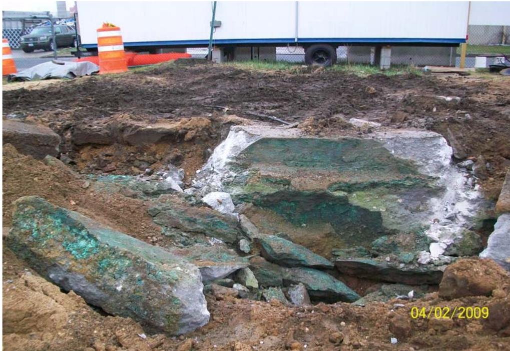
100\_00314.jpg - Green contaminated concrete on east foundation wall, looking east
