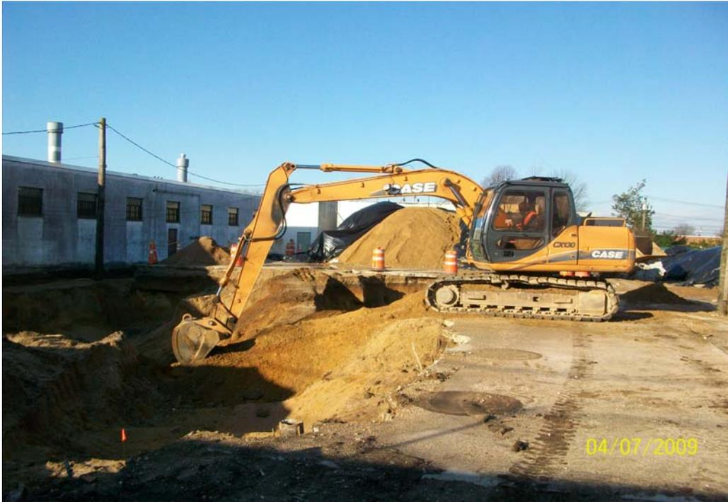
100\_00333.jpg - Excavator excavating ramp that was used to get to SEB-3/SES-5 area
