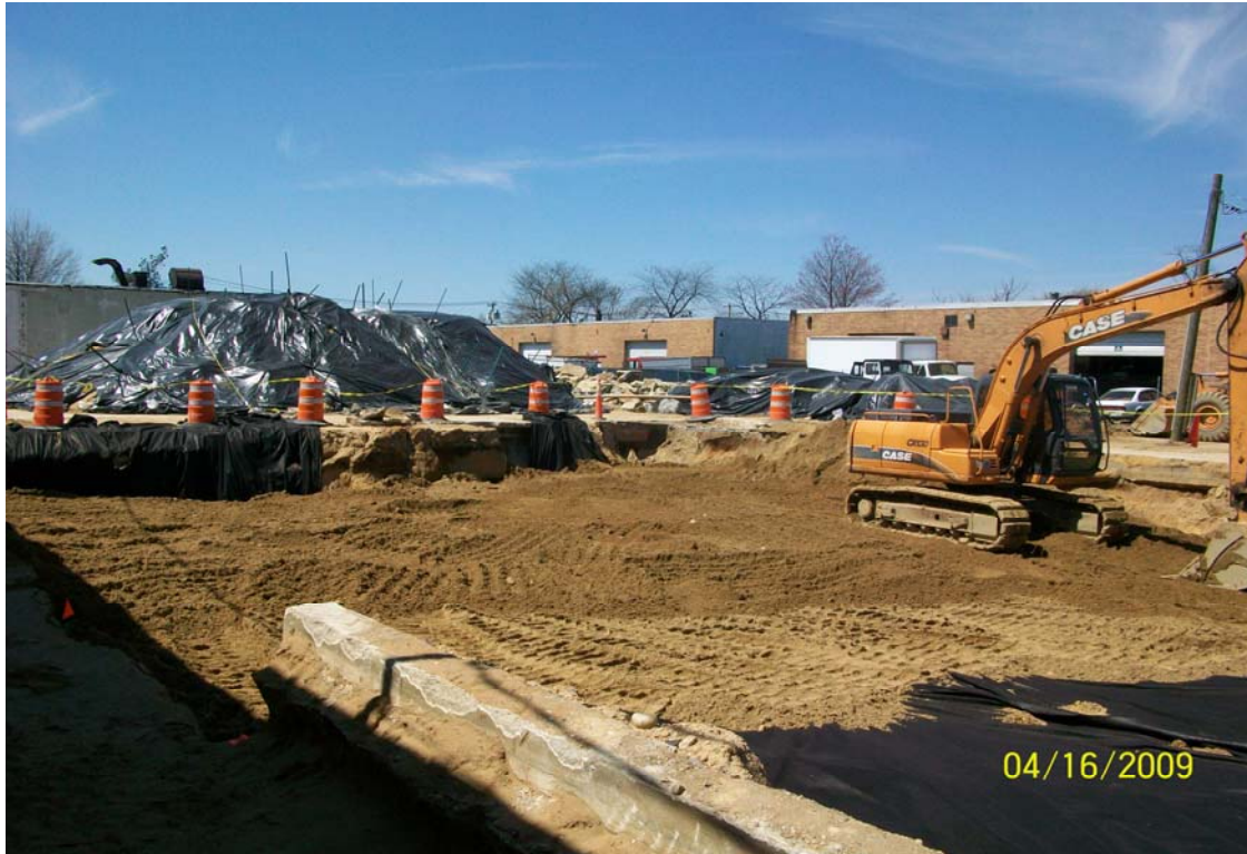
100_00375.jpg - Excavation at the end of the day, looking NW.
