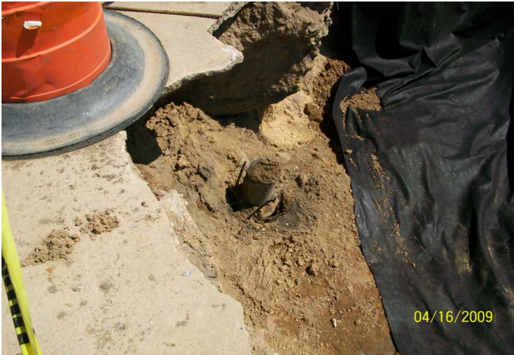
100_00373.jpg - Fire main pipe cut down below grade.
