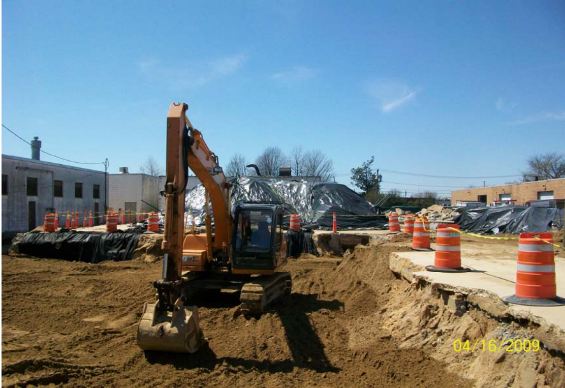
100_00376.jpg - Excavation at the end of the day, looking west.
