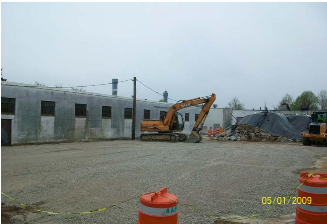
100\_00536.jpg - Compacted RCA to grade on the excavation at the end of the day, looking SW
