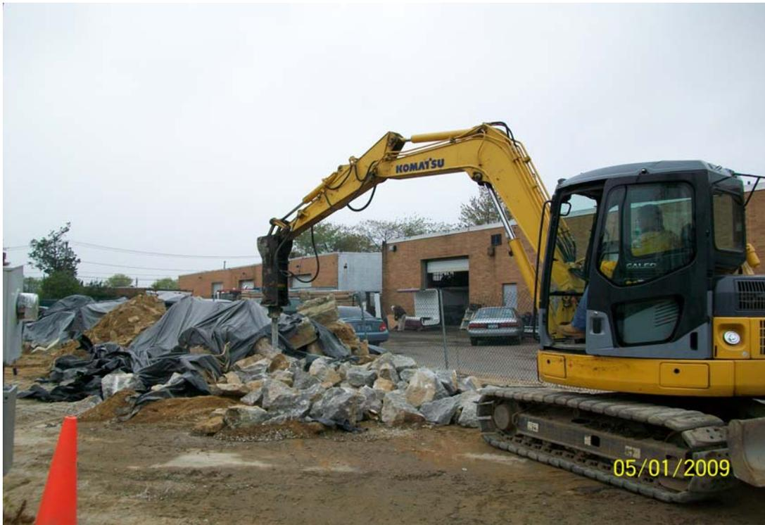
100\_00535.jpg - Breaking up concrete for disposal, looking NW
