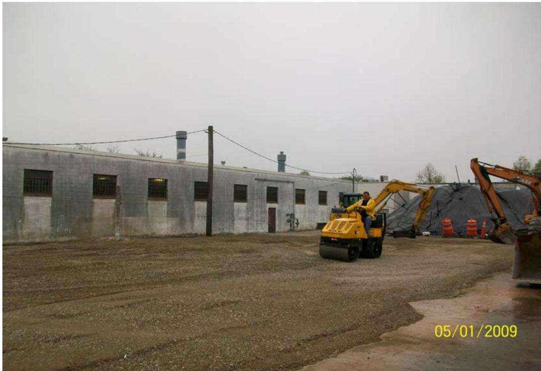
100\_00534.jpg - Compacting RCA to grade on excavation, looking SW
