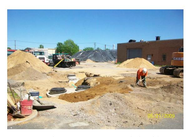
100\_00664.jpg - Septic system #1 partially backfilled (61 Cabot St.)
