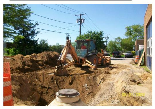
100\_00663.jpg - Septic system #4 partially backfilled (51 Cabot St.)
