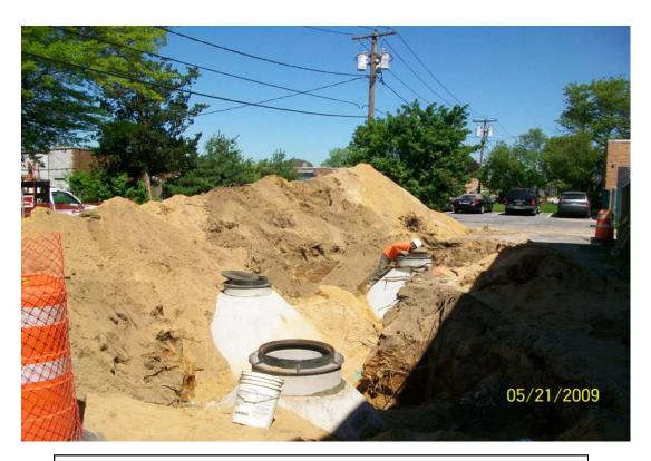
100\_00652pg - Completed septic system #4 (51 Cabot St.)
