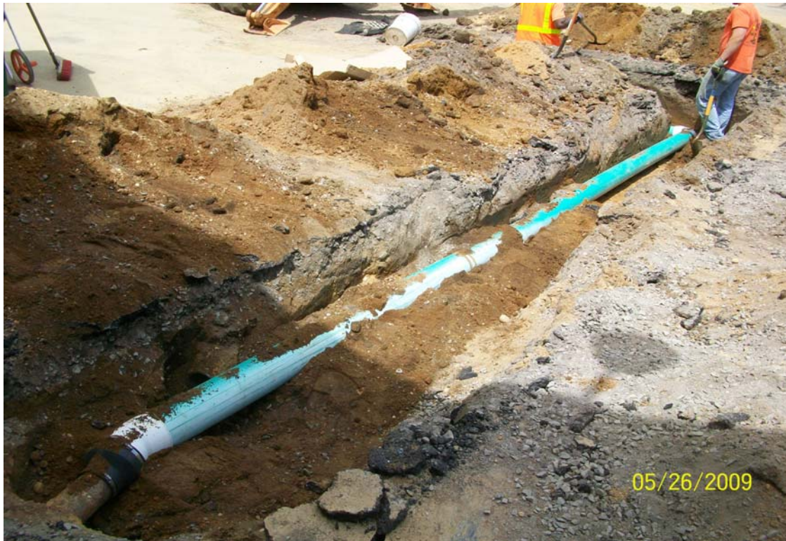
100_00685.jpg - Installing new roof drain piping to PDS-7, 51 Cabot St.
