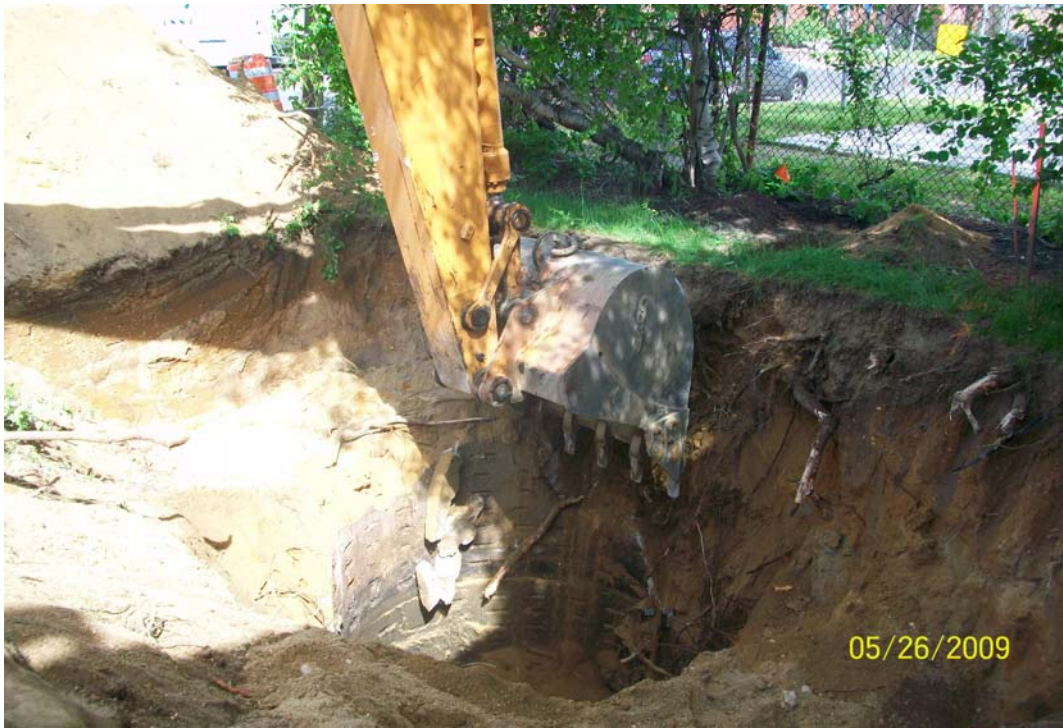
100_00681.jpg - Removing existing CP-13, 61 Cabot St.
