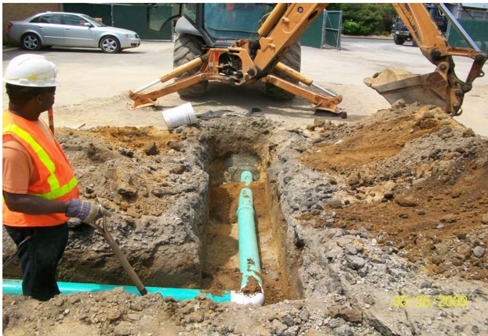
100_00686.jpg - Installing new roof drain piping to PDS-7, in background
