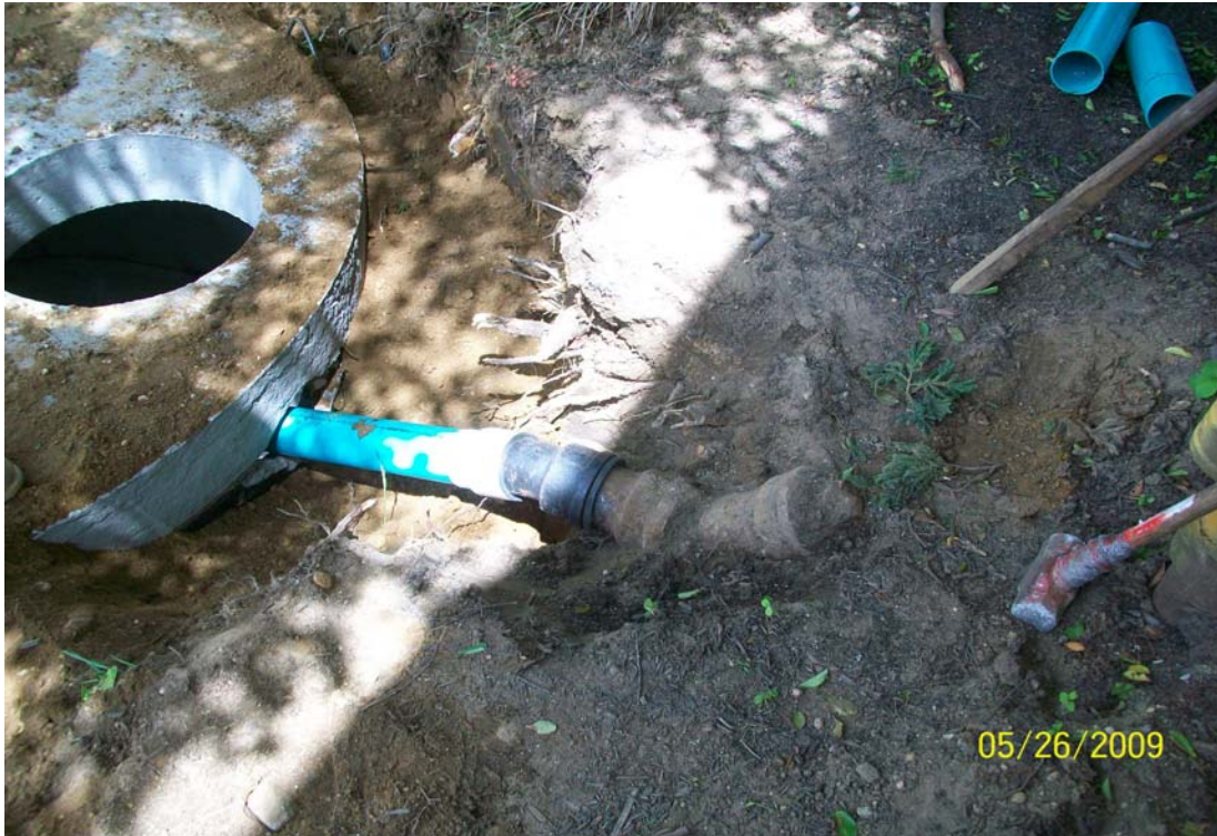
100_00684pg - Piping installed from 61 Cabot St. to PST-2
