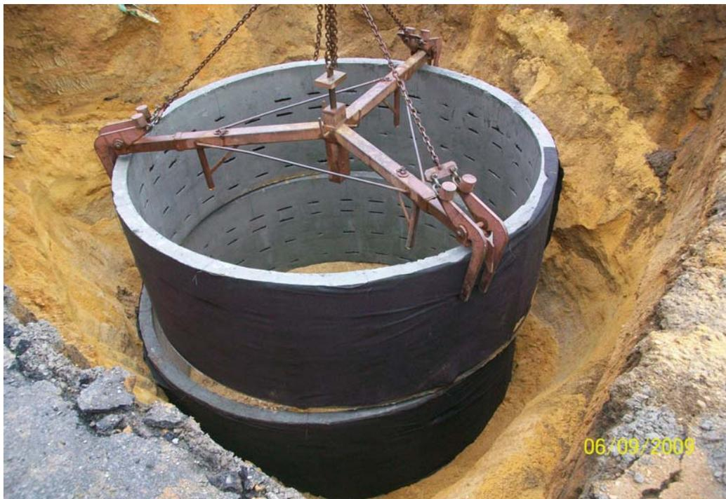
100\_0782.jpg - Installing PDS-9 structures wrapped in filter fabric, 60 Dale St.
