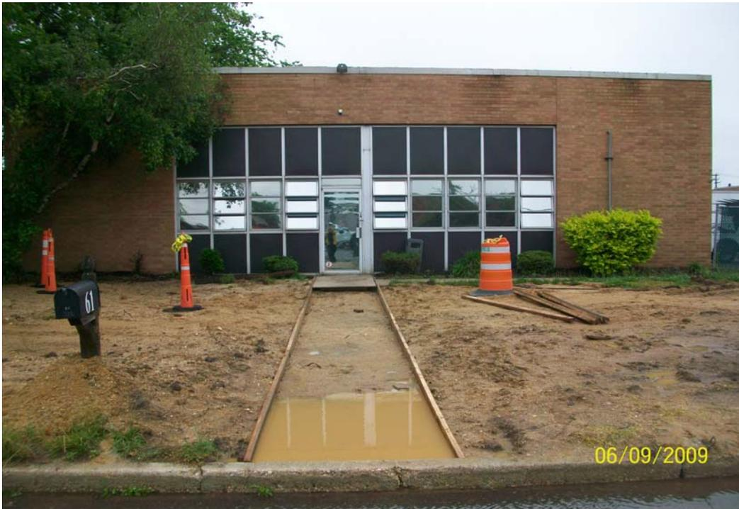
**100\_0784.jpg - Forms installed for replacement sidewalk in front of 61 Cabot St.**
