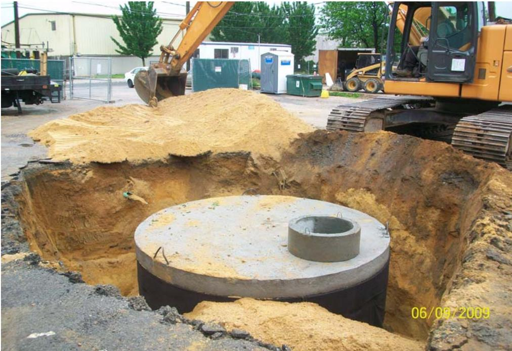
**100\_0785.jpg - PDS-9, 60 Dale St., being backfilled**
