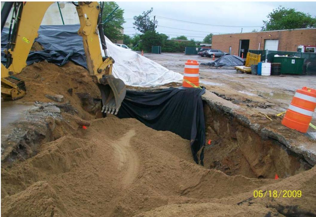
100\_0845.jpg - Starting to backfill and compact UST-5/9 excavation
