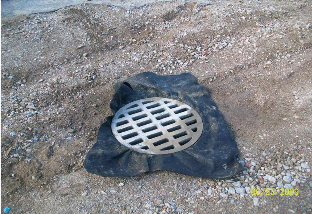
100\_0854.jpg - New filter fabric installed on new drainage structure cover
