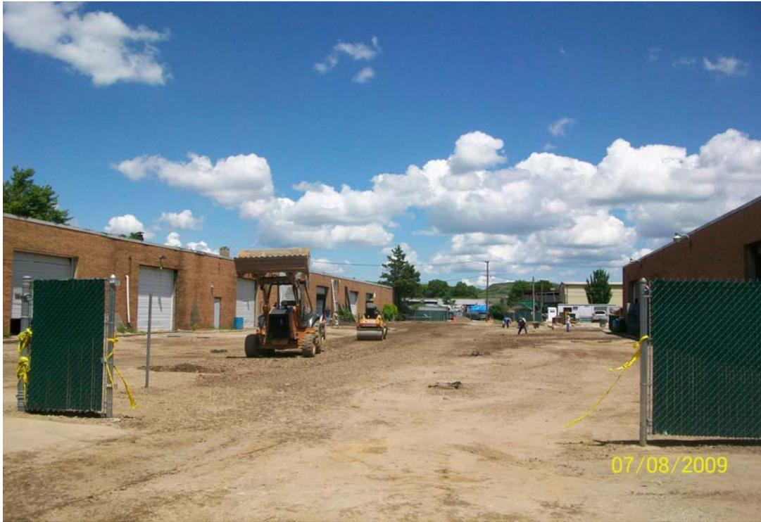
**100\_0941 - Accurate Blacktop grading and compacting RCA, looking east**
