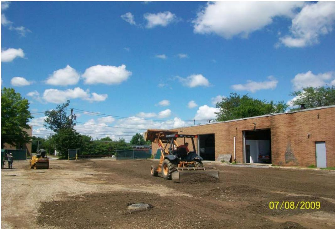
**100\_0940.jpg - Accurate Blacktop spreading RCA at 61 Cabot St.**
