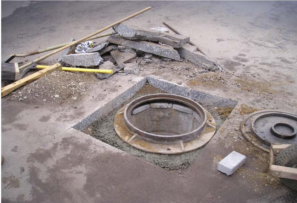
**P1010006.jpg - CP-3B cover re-installed and level with existing asphalt**
