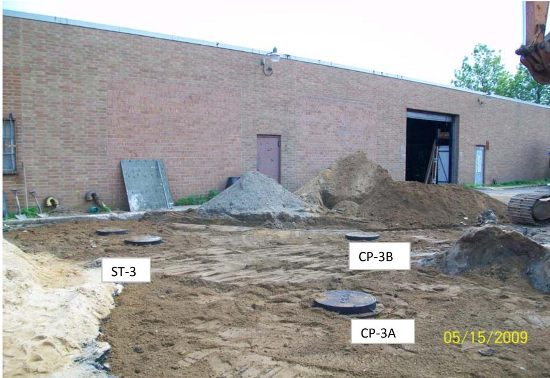
100\_0613.jpg - Completed installation of septic system #3, 51 Cabot St.
