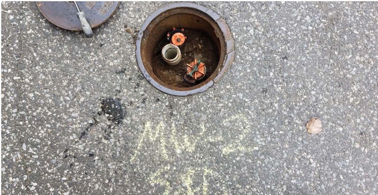
Photograph 10: Monitoring well manhole containing MW-02S & MW-02D.
