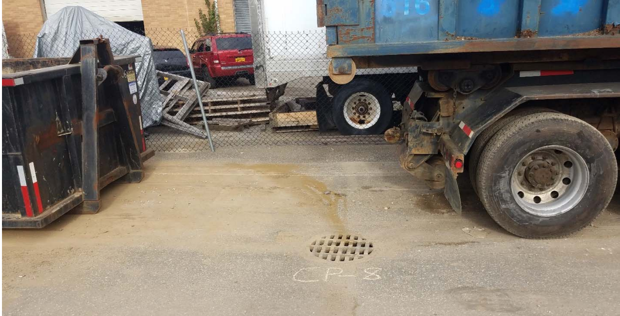
Photograph 5: Restricted excavation location for cesspool, CP – 8. No apparent subsurface disturbances noted in accordance with restricted use.
