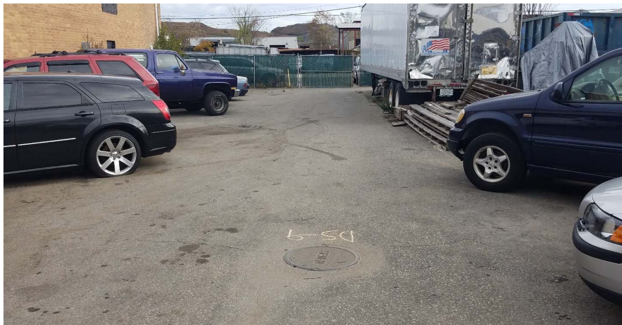
Photograph 8: Restricted excavation location drainage structure, DS – 9. No apparent subsurface disturbances noted and in accordance with restricted use.
