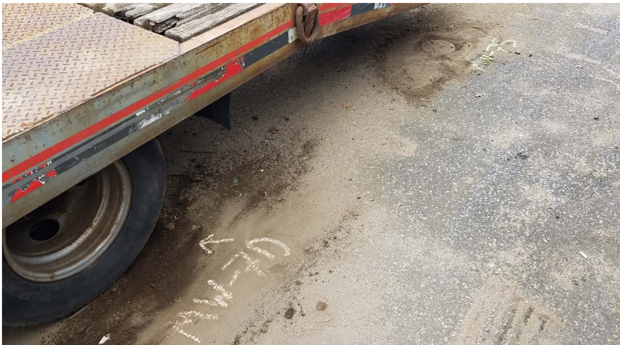
Photograph 14: Monitoring well manhole locations for MW-07D (lower-left) & MW-01S (upper-right).
