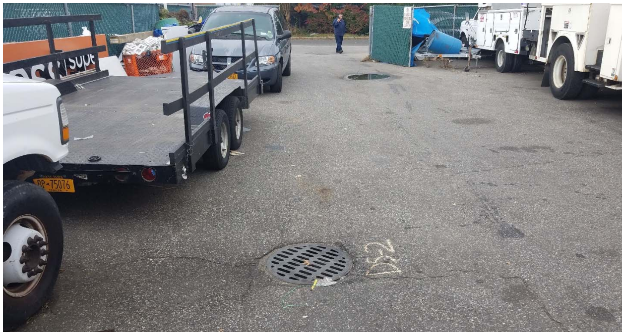
Photograph 2: Restricted excavation location for drainage structure, DS – 2. No apparent subsurface disturbances associated with this drainage structure location.
