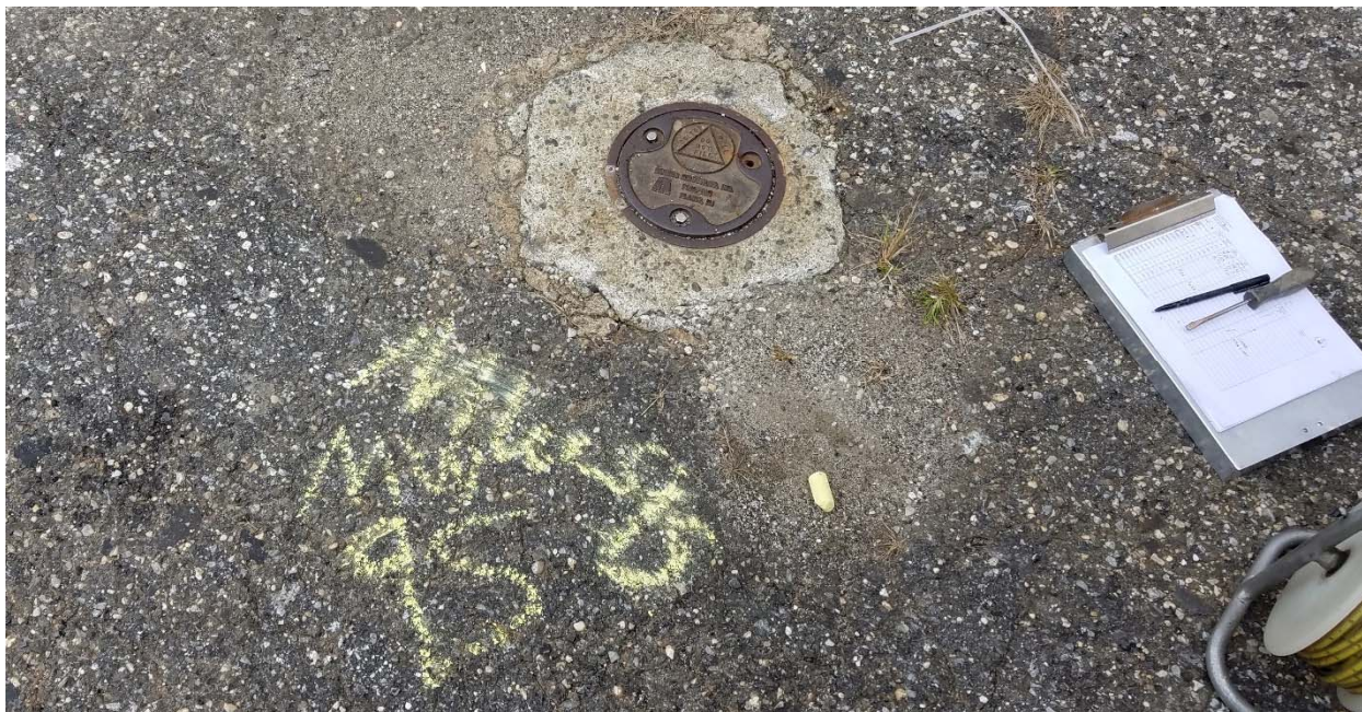
Photograph 15: Monitoring well manhole location for MW-09S.
