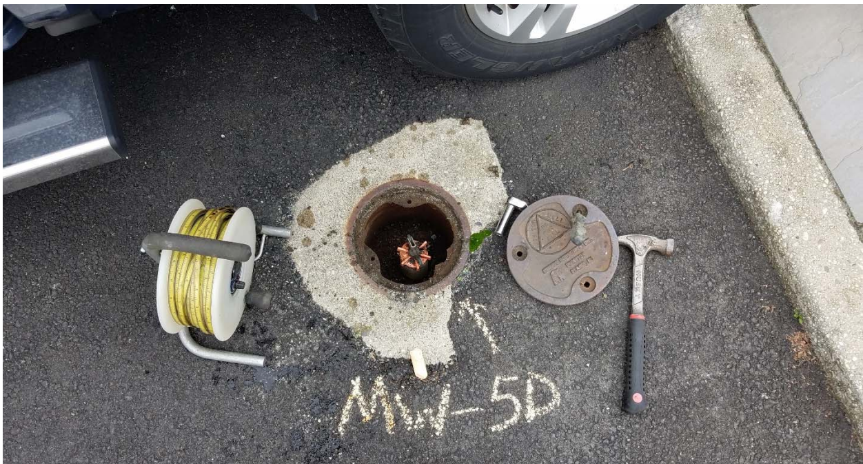
Photograph 12: Monitoring well manhole containing MW-05D.
