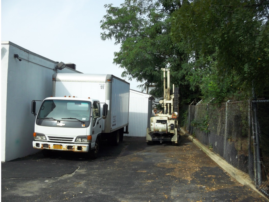
Installation of TW-3
