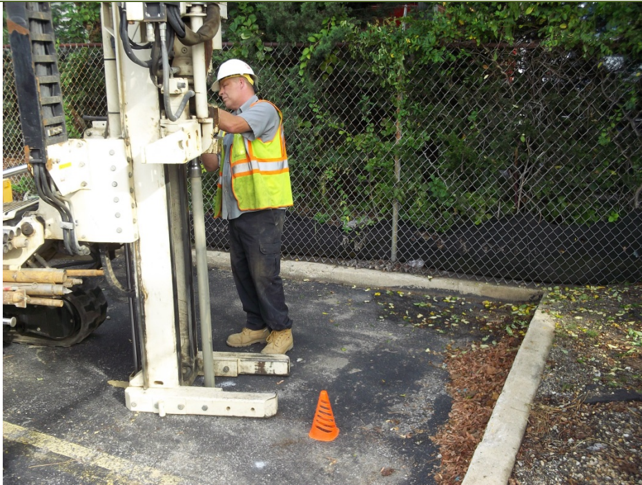
Installation of TW-2
