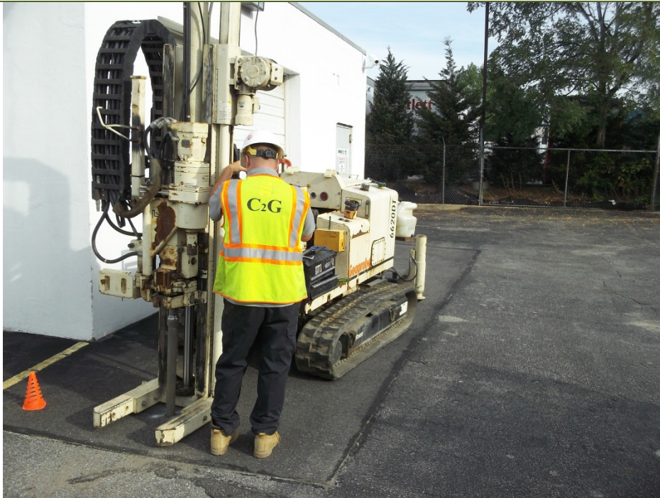
Installation of TW-1
