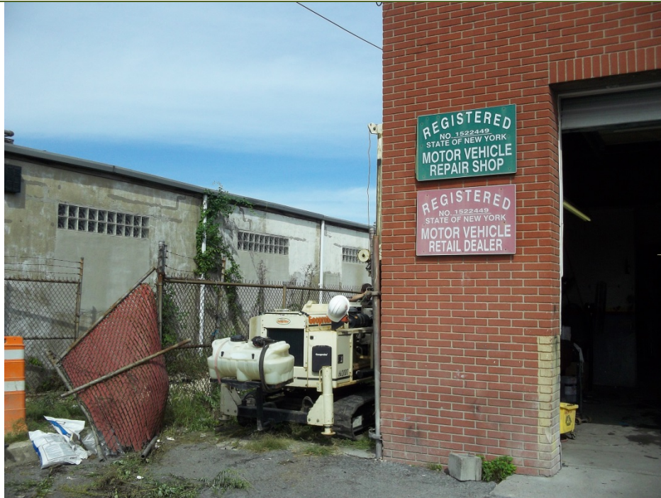
Installation of TW-5
