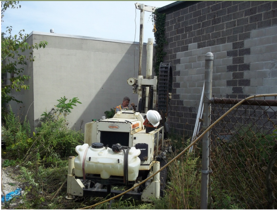
Installation of TW-4
