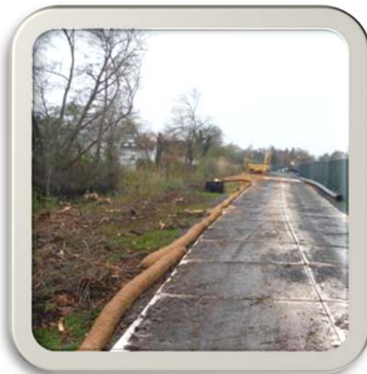
Straw wattles being used for erosion control
