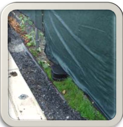
Rodent control device inside construction fencing with privacy screen
