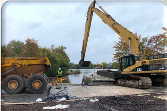
Offloading lake sediment from scow for transport to TFS
