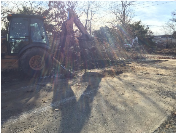
The start of excavation of SB-18, viewed to the southeast.
