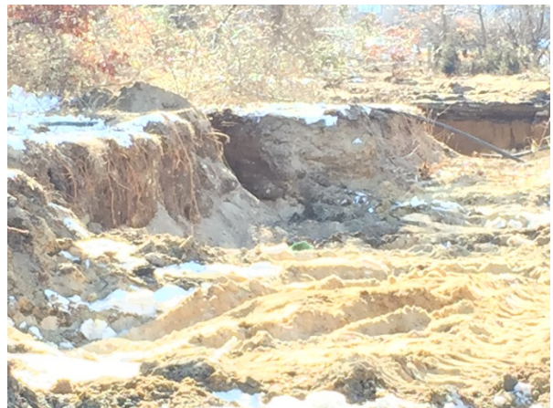
The final extents of location SB-22/18/19-S2. Excavation ceases and the area remains devoid of backfill.
