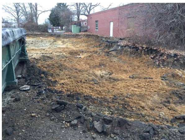
Overview of the SB-22/18/19 excavation, viewed to the west.
