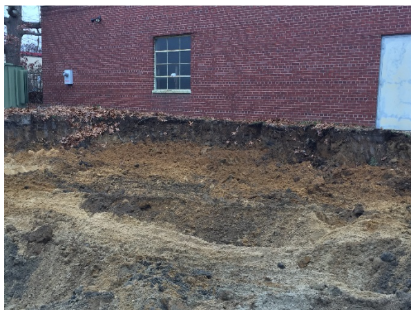
Petroleum-like impacted soils are no longer observed to the north as the excavation nears the former Plastics Manufacturing Building.
