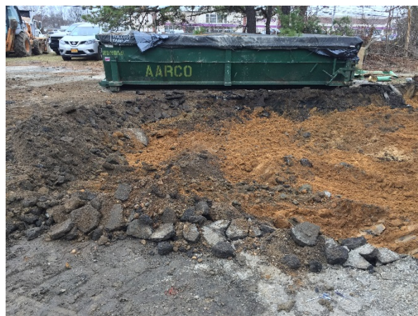
Petroleum-like impacted soils are no longer observed to the east as the excavation nears the main building, viewed to the south.
