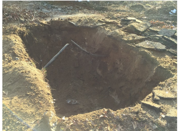
Excavation of SB-22, viewed to the south.
