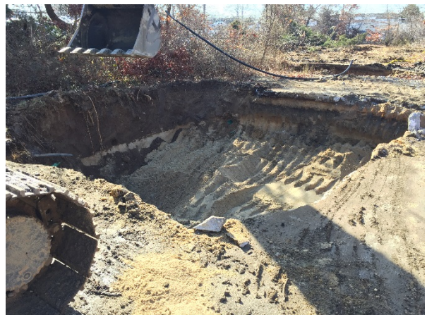
Excavation of SB-18 extends further north to find the extents of the impacted soil, viewed to the southwest.
