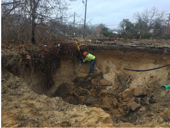
Endpoint sampling of sidewall SB-22/18/19-S1 is conducted, viewed to the south.
