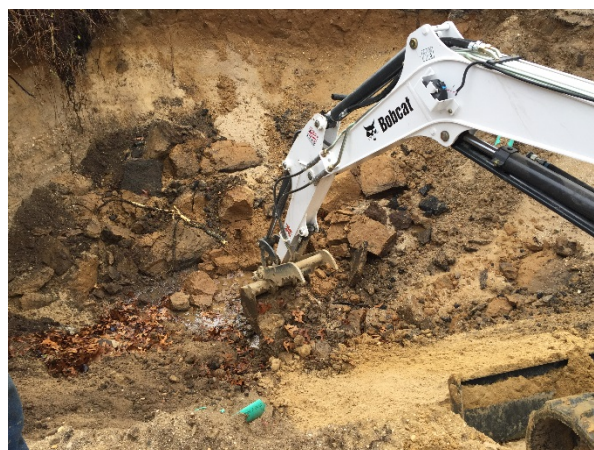
Impacted soil is removed from SB-22 and a layer of sand is reached at approximately 8'.
