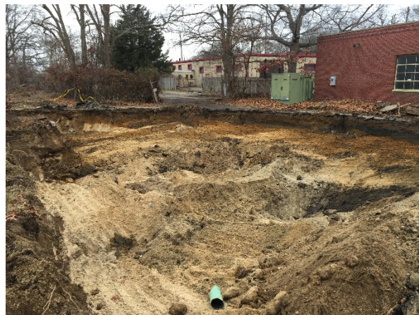
Impacted soils are removed from select locations where the contamination extended deeper than 4'.
