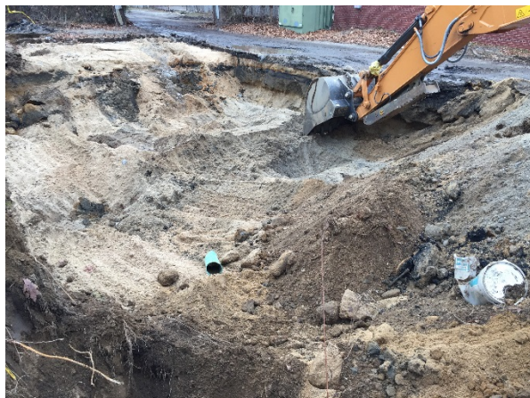
The excavation of SB-18 combines with the excavation of SB-19 due to the areas where impacted soil is found, viewed to the northwest.
