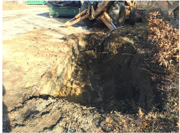
Excavation of SB-18, viewed to the east.
