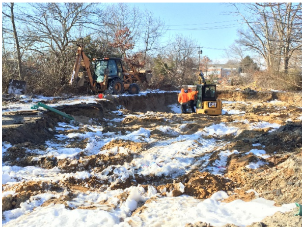
Sidewall sample SB-22/18/19-S2 exceeded the Part 375 SCOs for cadmium. The sampling location was excavated further and resampled.
