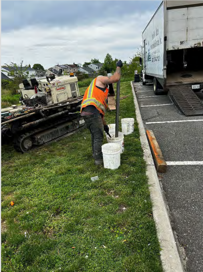
LAWES decontaminating drilling steel.
