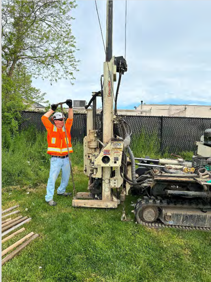
Drilling subcontractor (LAWES) hand-clearing ISB-B3 boring prior to drilling.
