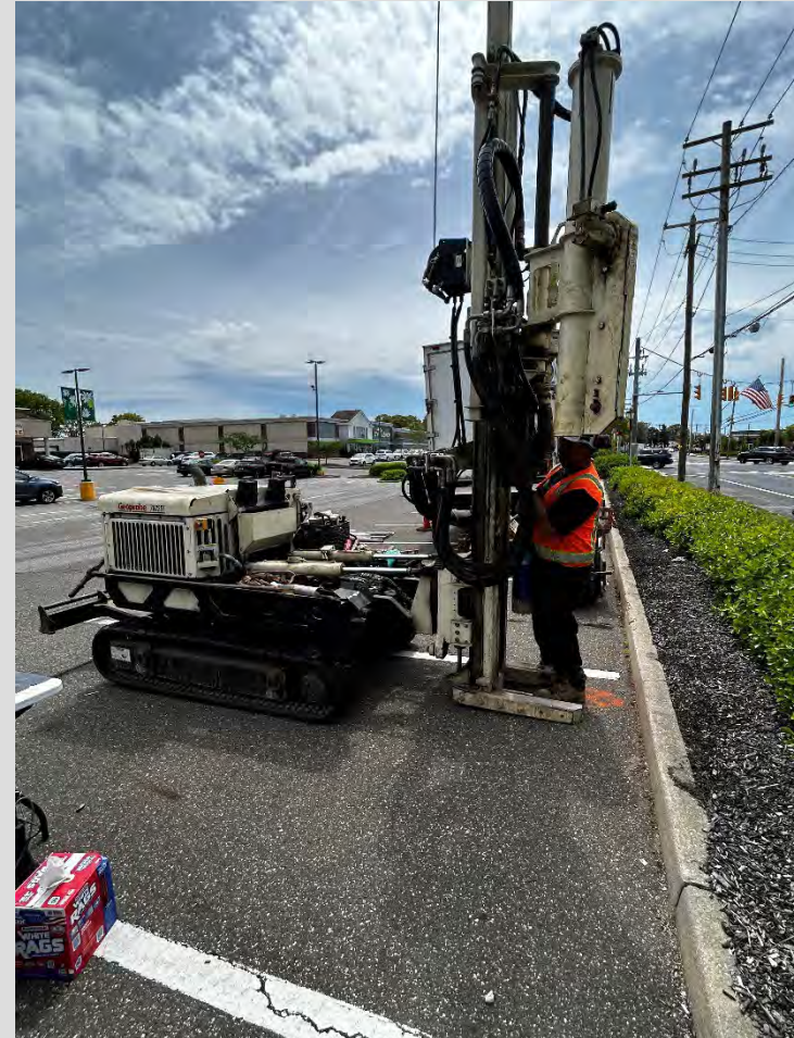
LAWES coring through asphalt at ISB-A4 Location.
