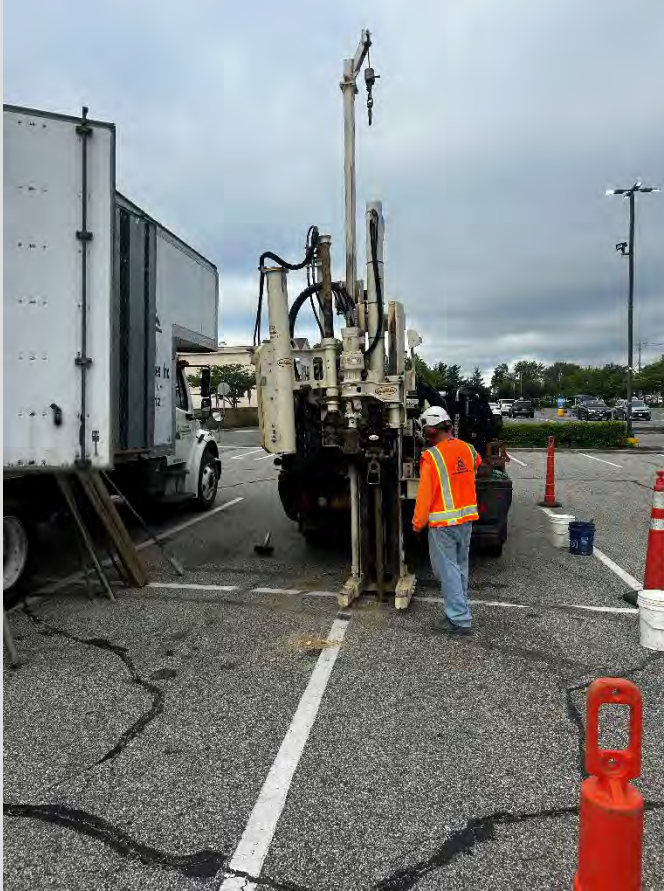
LAWES advancing ISB-C2 boring with Geoprobe rig.
