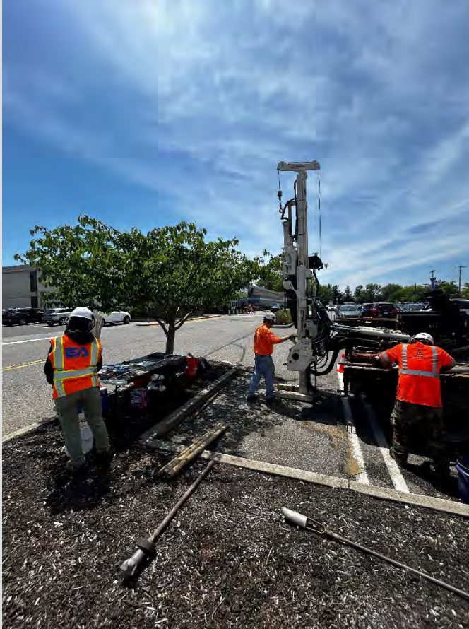
LAWES advancing soil boring at ISB-C1 location with Geoprobe.
