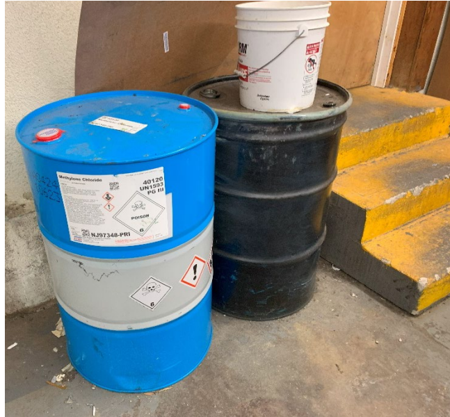
Above: Representative view of the concrete building slab in a chemical storage area on the first floor of the building. The drums include virgin methylene chloride and waste ink (black drum). No spills or evidence of releases was noted and the concrete was observed to be intact throughout this area, with much of its surface painted or coated.
