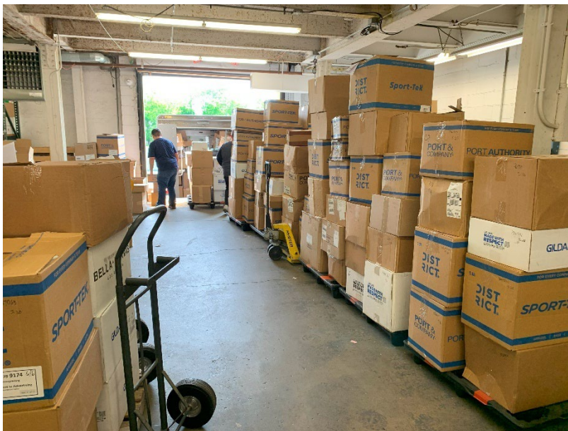
Above: Another representative view of the concrete building slab in the shipping area on the first floor of the building. The concrete was observed to be intact throughout the first floor, with much of its surface painted or coated.
