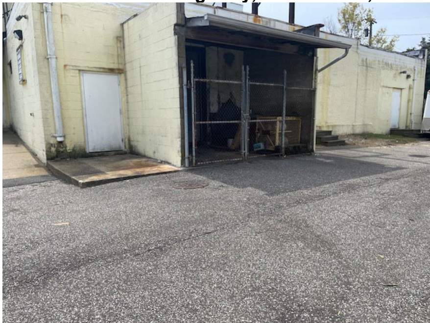
Above: View of the rear of the onsite building and part of the asphalt pavement cover over the former LP-1 area (far right). The pavement was observed to be in good condition throughout the covered area.
