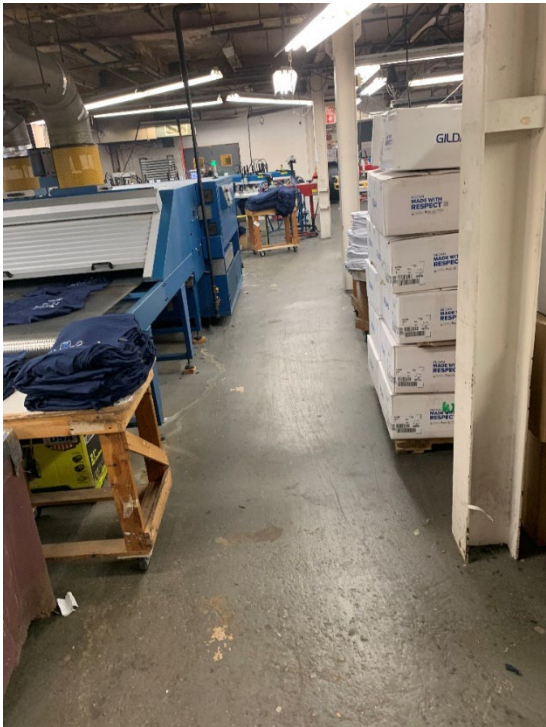
Above: Representative view of the concrete building slab in the manufacturing areas on the first floor of the building. The concrete was observed to be intact throughout the first floor, with much of its surface painted or coated.
