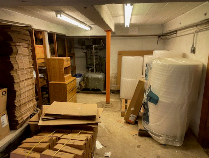
Above: Representative view of the concrete building slab in the basement, which underlies a portion of the building and is used solely for storage and utilities. The concrete was observed to be intact and in good condition throughout the basement.
