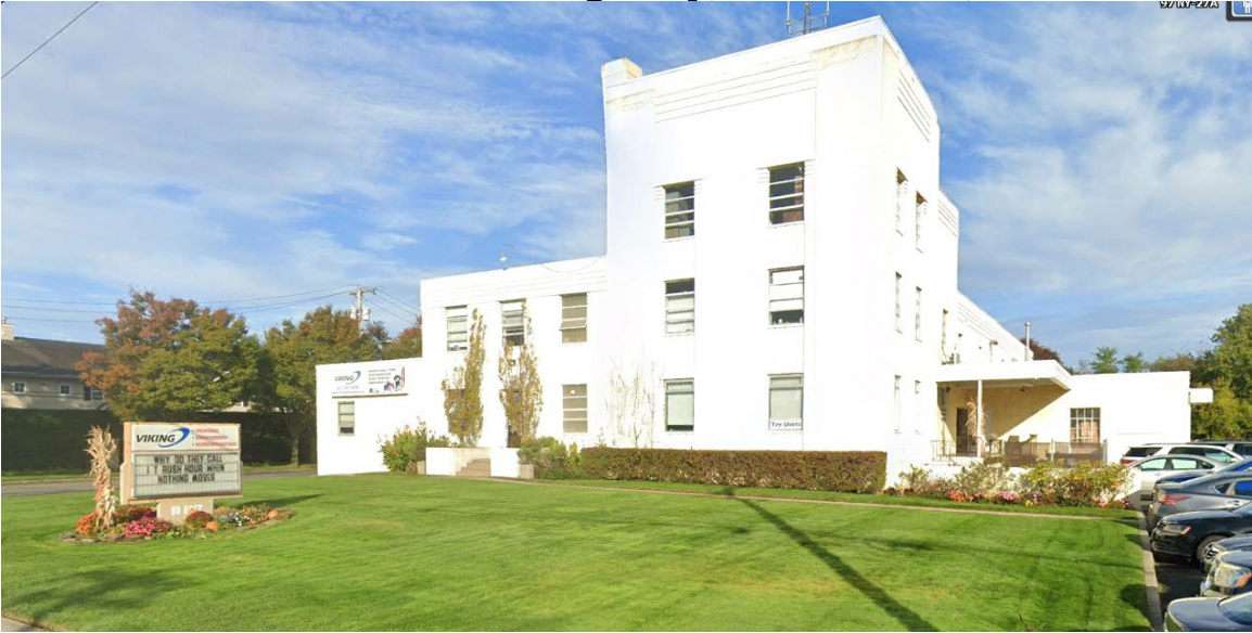
Above: View of front (south side) and part of east side of the industrial building at the subject property looking north.
