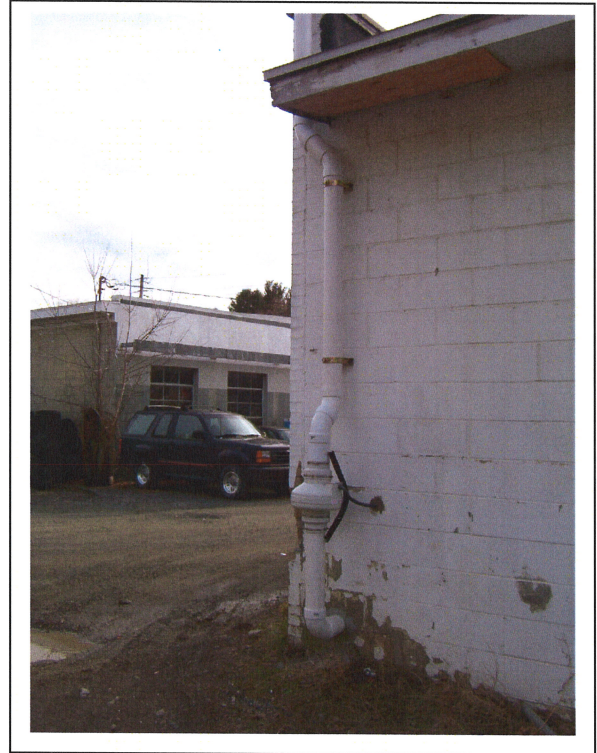
Photo #6: Blower for extraction points along southeast wall.
