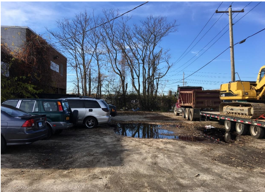
Photo showing parked vehicles, disposal truck and excavator in front of the site building:
