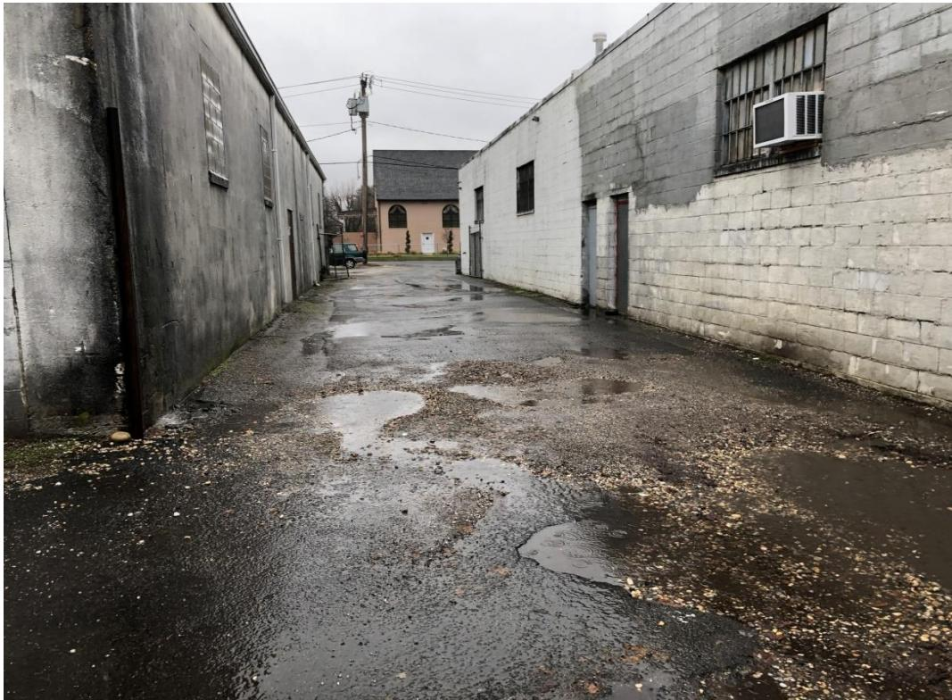
Photo showing parked cars at the south of the site facing west (pondings at uneven asphalt pavement):
