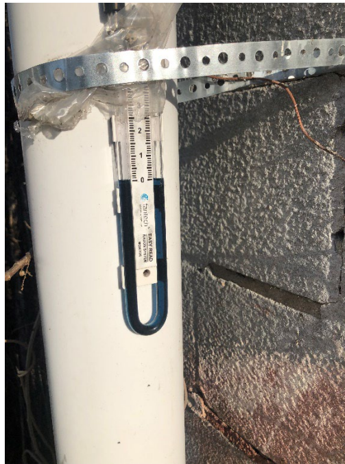
U-tube manometer on SSDS
