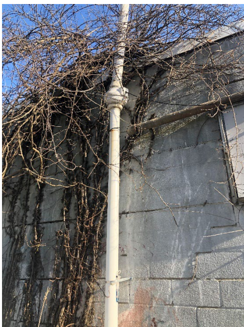
Offline SSDS (radon fan)
