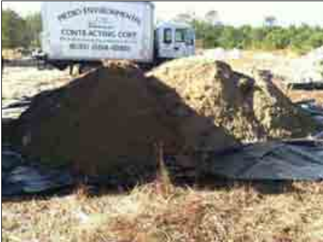
Photo 13 – Soils stockpiled on polyethylene sheeting in staging area.
