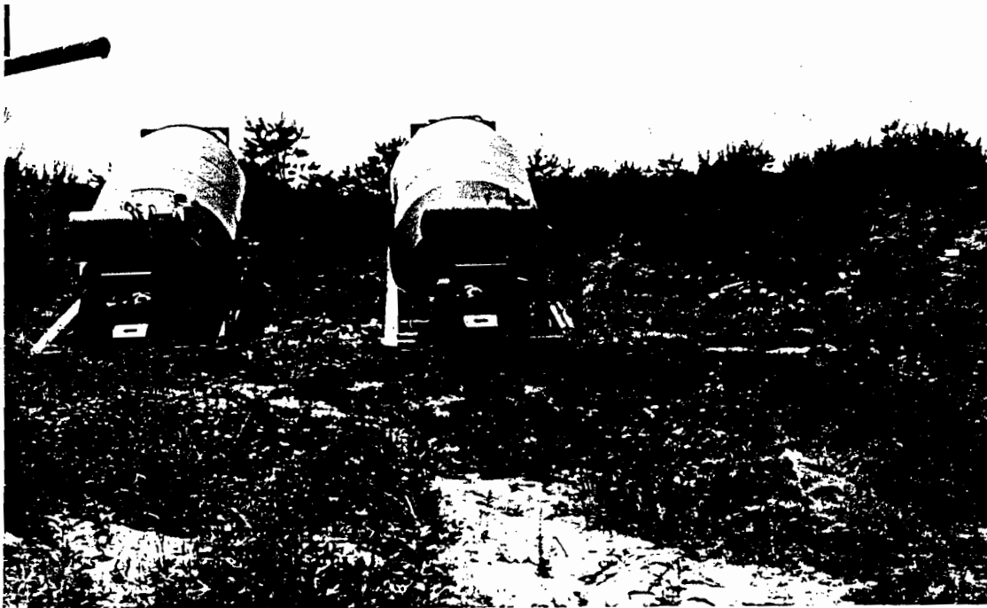
FACING WEST - TWO CONCRETE MIXERS AND OTHER ABANDONED MACHINERY.
