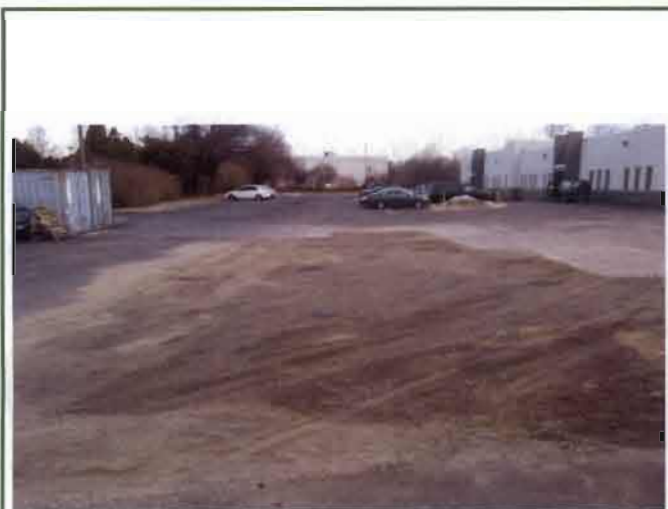
Photo #7 – View of the completed work area looking north.
