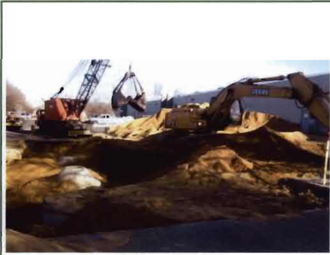
Photo #6 – View of the new leaching pool being backfilled. LP-1R is shown in the foreground, LP-3R in the background.
