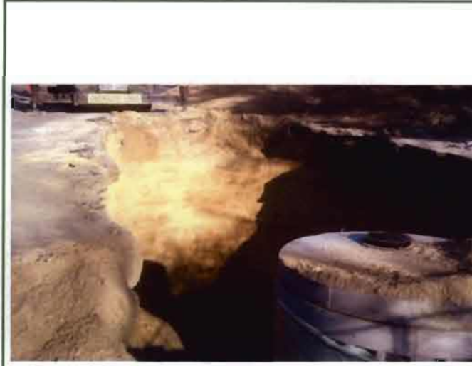
Photo #2 – View of LP-1R and the excavation for LP-2R.
