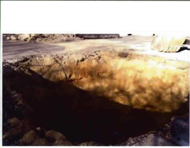
Photo #1 – View of the excavation for LP-1R.
