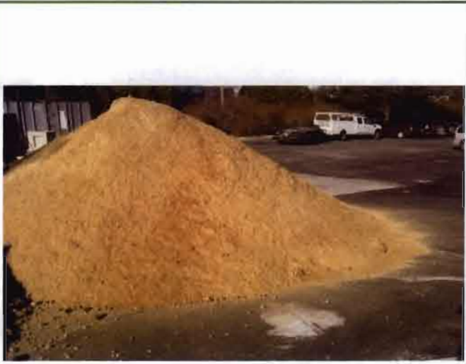
Photo #5 – View of the stockpiled material excavated during the installation of LP-1R through LP-3R.
