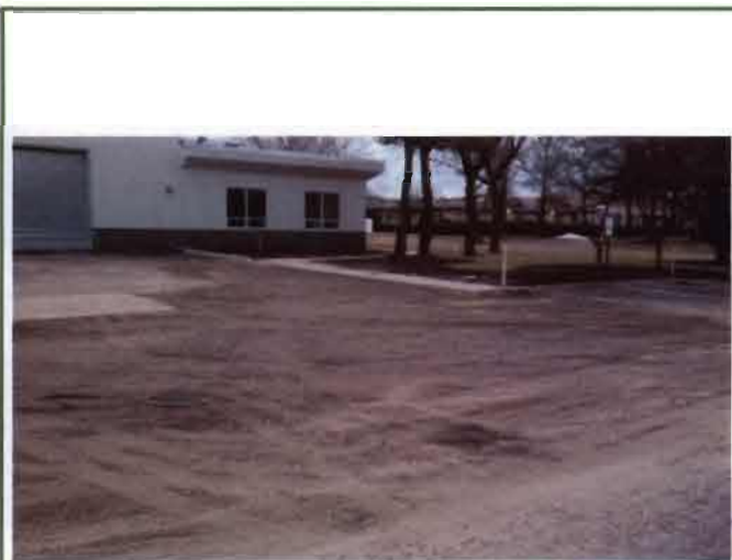
Photo #8 – View of the completed work area looking southeast.
