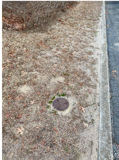
Above: Monitoring well MW-16 at the northwest corner of the Site. The condition of this monitoring well (intact, manhole cover in place) is representative of the other monitoring wells.
