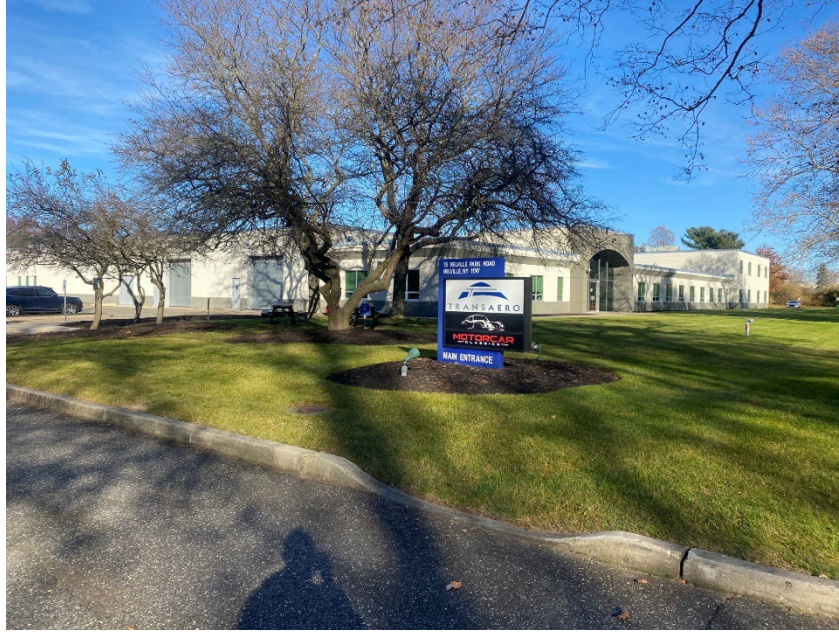
Above: A view of the front of the Site from the southwest corner.
