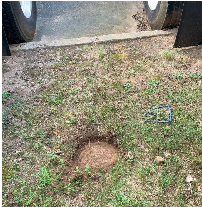
Above: Monitoring well MW-5 on the west side of the Site. The condition of this monitoring well (intact, manhole cover in place) is representative of the other monitoring wells.
