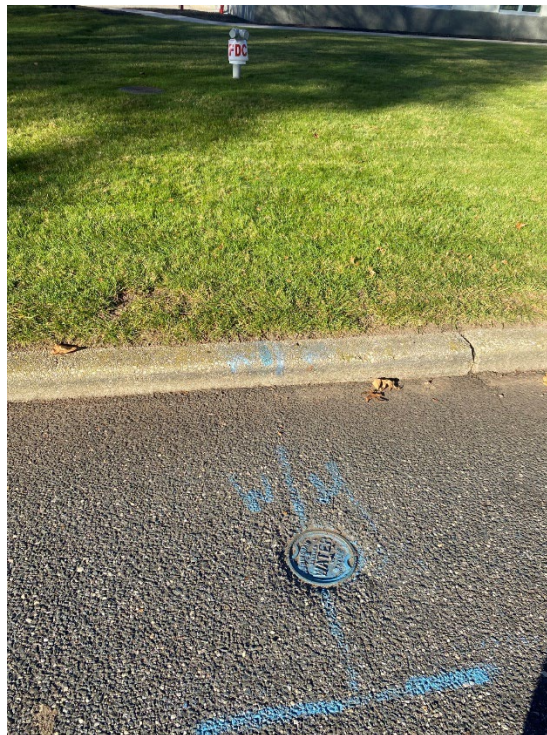
Above: Public water connection on the Site.
