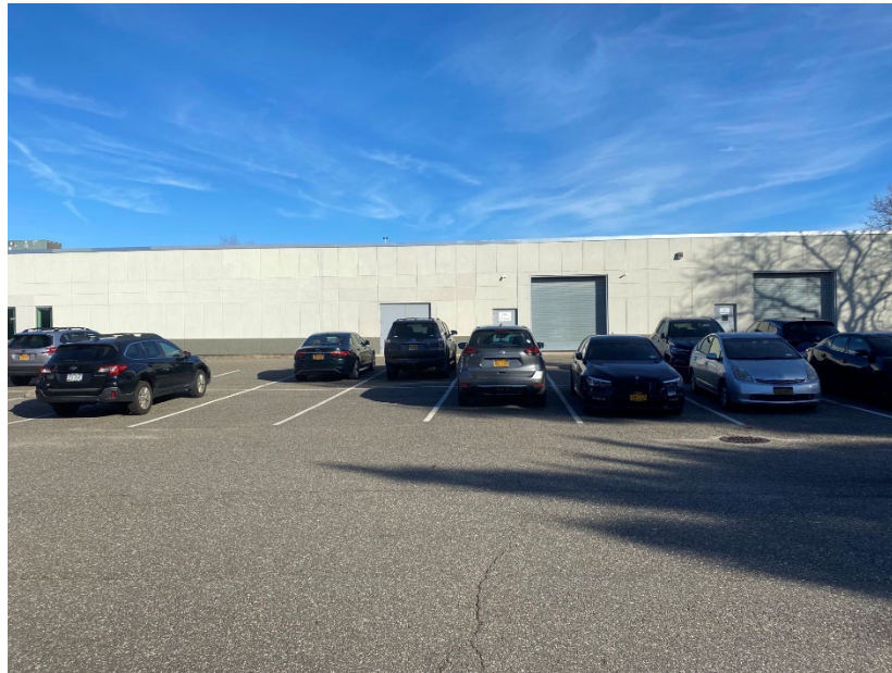
Above: Intact pavement featuring no new disturbances above cover over former leaching pool LP-3.
