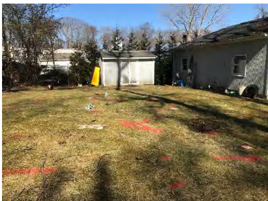
107 Laurel Ln S-N: Photo of the site location containing 19 soil borings in total going South to North. The pink lines shown above illustrate unknown utilities that were found.
