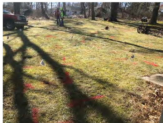
107 Laurel Ln N-S: Photo of the site location containing 19 soil borings in total going North to South. The pink lines shown above illustrate unknown utilities that were found while the few red lines show power tones that were found.
