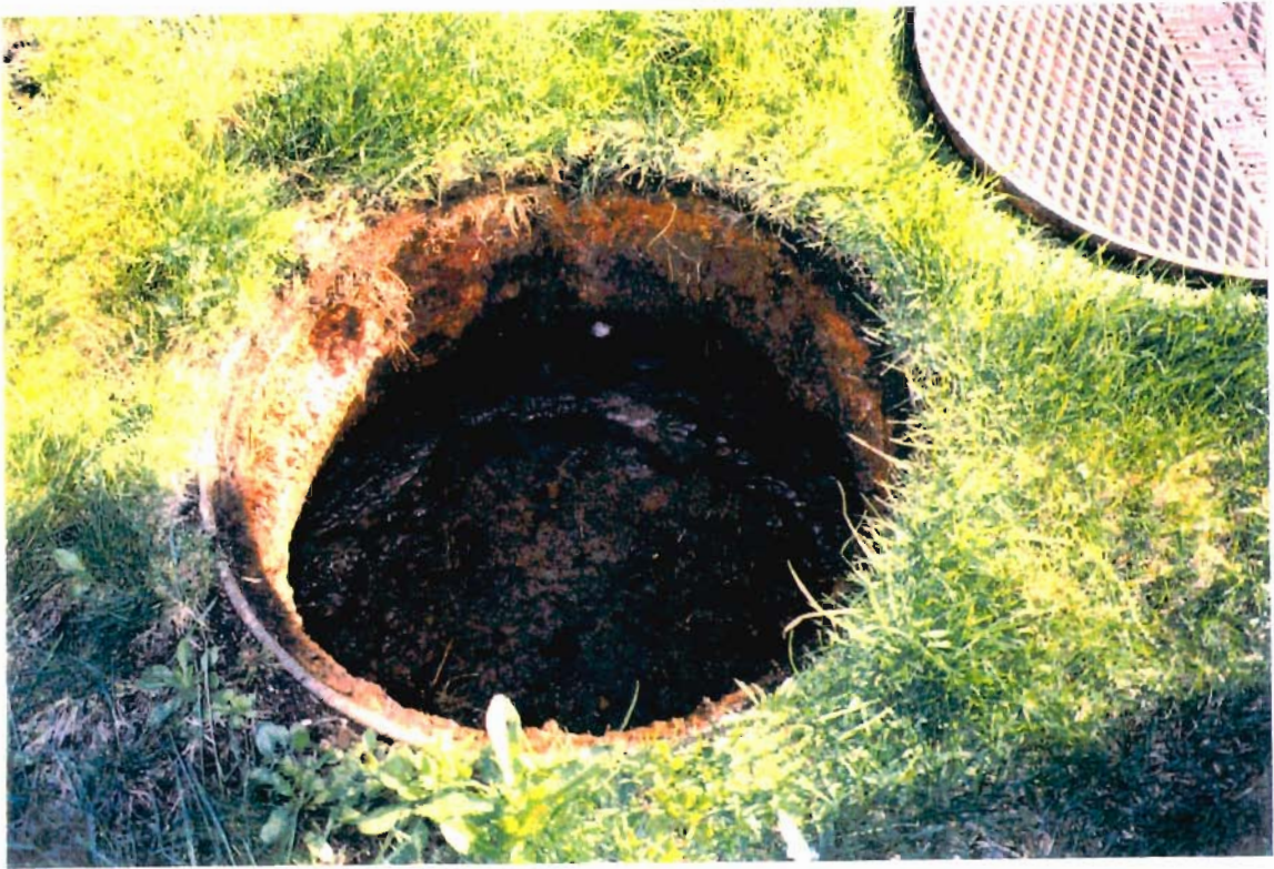
SEPTIC TANK BEFORE CLEANOUT
