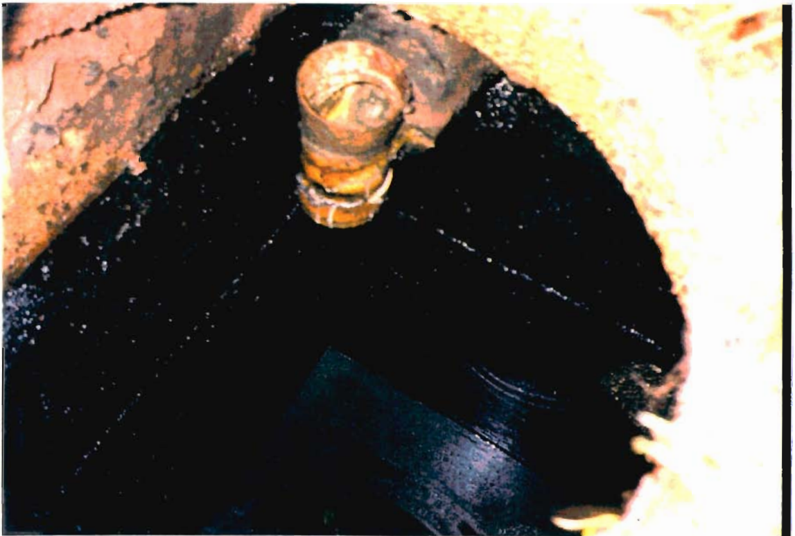
SEPTIC TANK AFTER CLEANOUT
