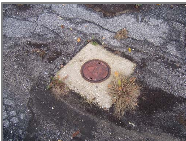
MW-3: a well in good shape. Note the round white pebbles in the concrete apron. More to say about this later.
