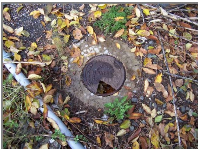
A well with a cracked cover
