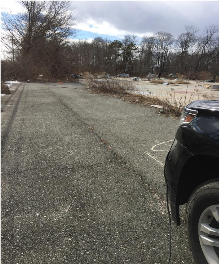
View of asphalt cap looking west
