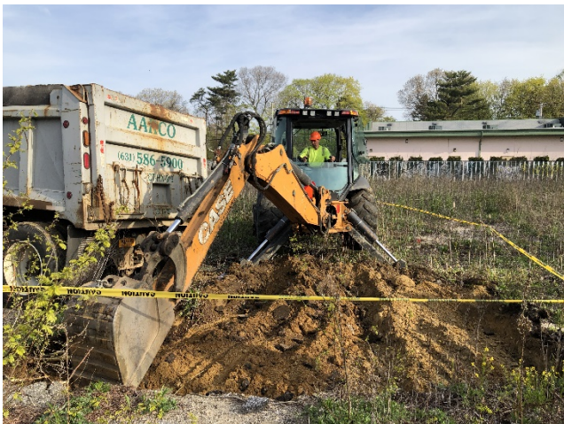
Photo 7: Excavation process in Area 1 with excavator.
