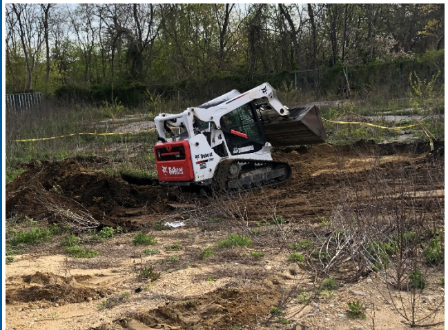
Photo 8: Excavation process with Bobcat compact track loader.
