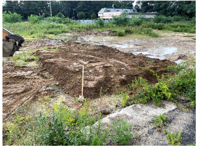
Photo 2: View of the capped area with one foot of clean soil cover.
