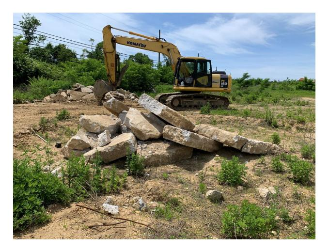
Below: Former temporarily-capped area after removal of additional soil from the north and south ends . This area is now approximately 20 feet wide, 35 feet long, and between 3 and 5 feet deep. View is looking south at the former foundation adjoining the abandoned tank area. Confirmatory samples were collected from the floor and north wall of the enlarged excavation.
